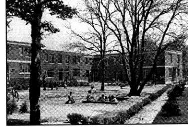
Fig 17.22 - Apartments - Chicago, Illinois
