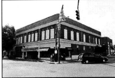
Fig 17.12 - Corner Fabric - Blacksburg, Virginia
