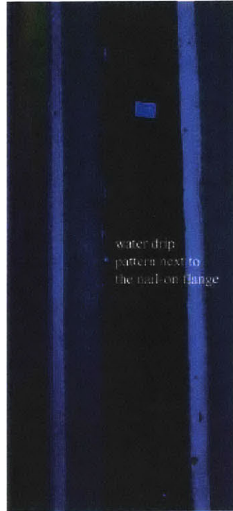
Figure 2-42 Test 13 drip pattern along the window jamb edge
