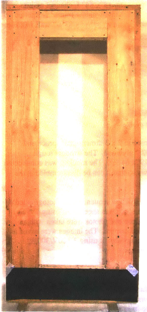
Figure 3-9 w-Flashing installation sequence - step 1
