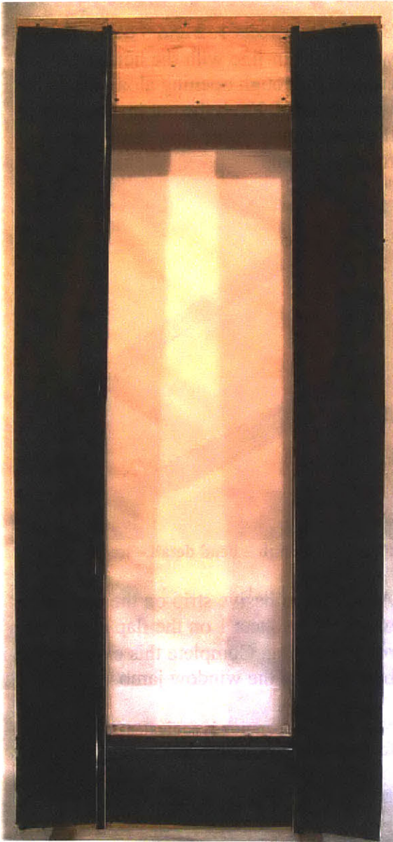
Figure 3-13 w-Flashing installation sequence – step 2
