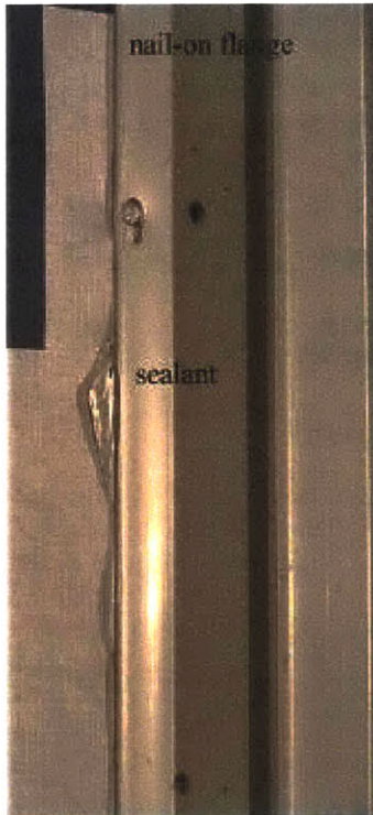
Figure 2-53 sealant applied in the lap joint
