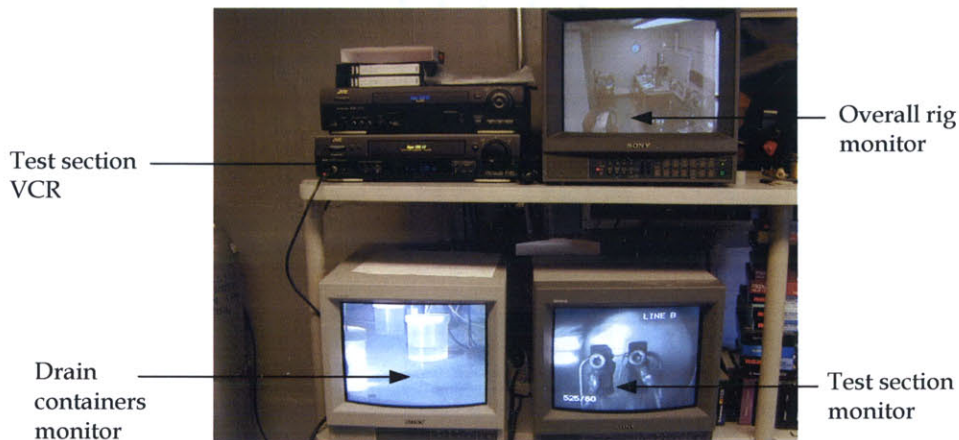
Figure 3-11: View of the right side of the control room.
