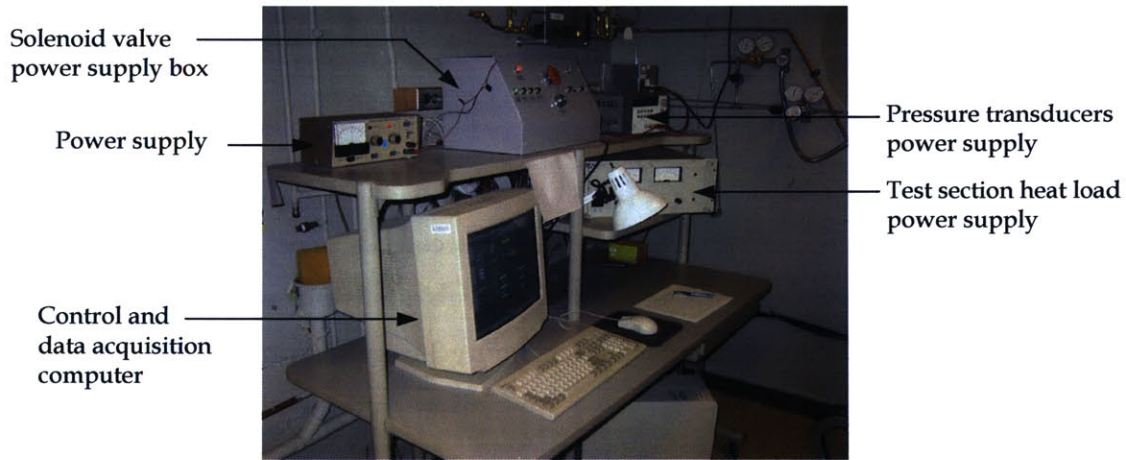
Figure 3-3: Left view of the control room.
