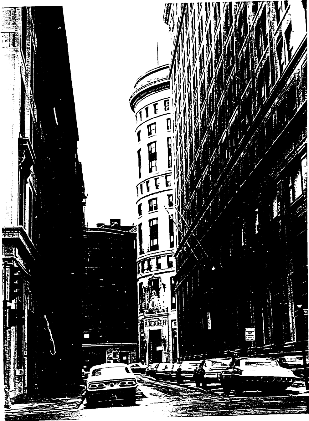
FIGURE 3.2: Building Surface Irregularities
