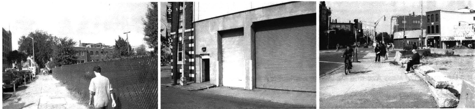
The current conditions of the sidewalks at Mass Ave around the MIT campus are deplorable.
