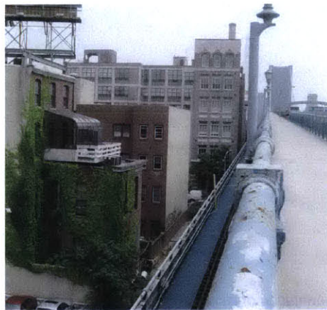
13 views of the rooftops, from the Benjamin Franklin (Delaware River) Bridge
