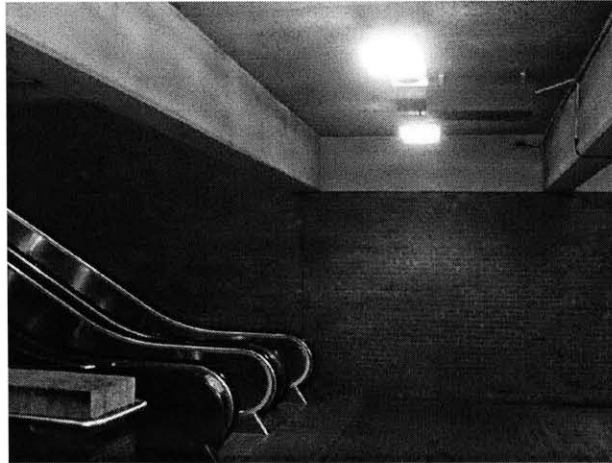
Figure 5-4: View of Davis system. The sign will be projected against the brick wall to the right of the escalators.
