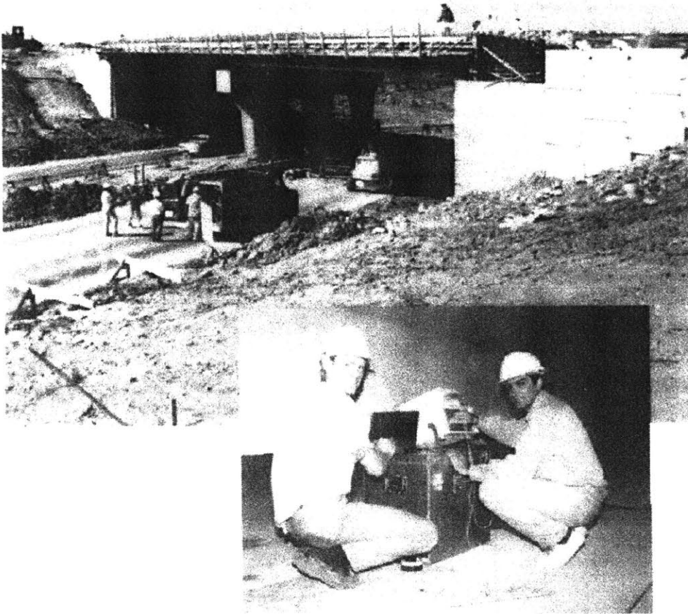
Figure 21: Beddington Trail Bridge (Top), a four channel Bragg grating demodulation system used (Bottom) (Measures et al., 1995)
