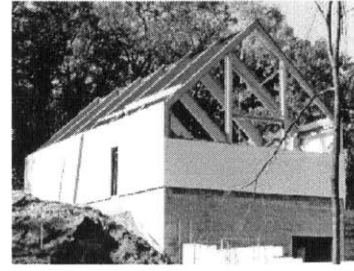
Amador Corp. Facility
