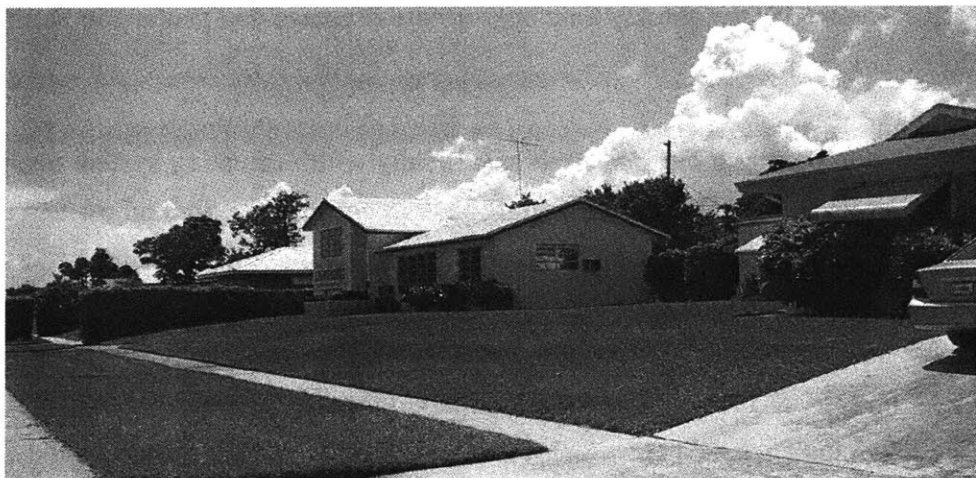
Fig. 68. Flood elevation, Roosevelt Estates, 2003
