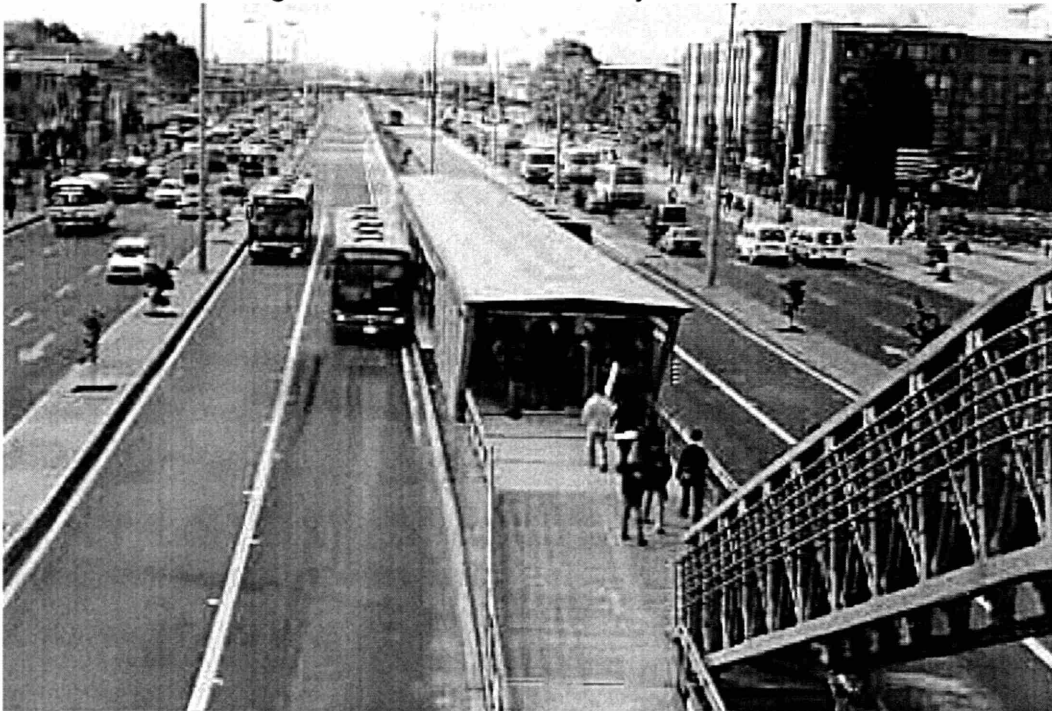
Figure 23. TransMilenio busway and station on 80 th Street
