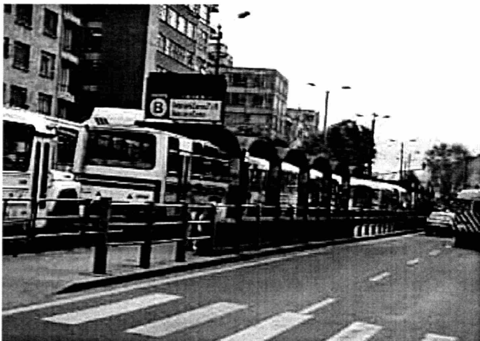
Figure 15. The Caracas Avenue busway in 1999, south-north direction.
