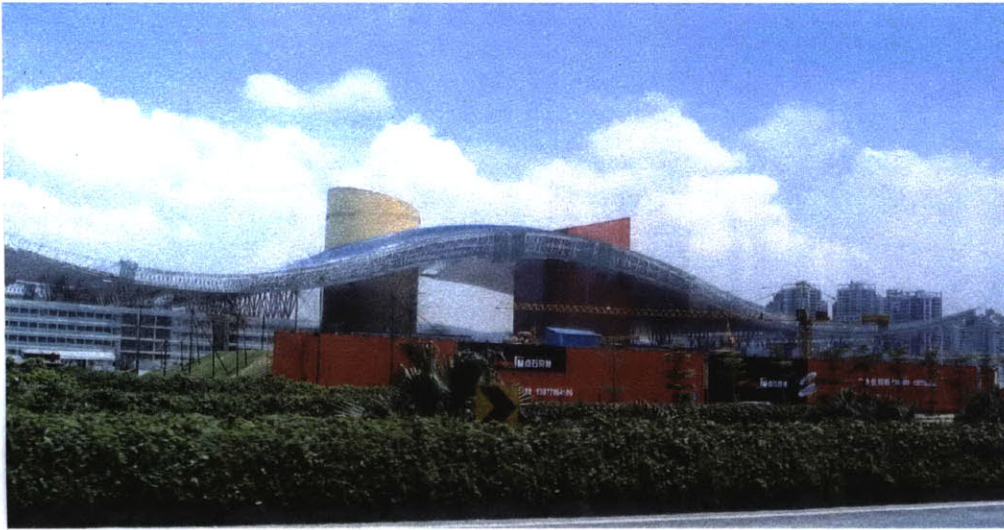
Figure 89. New Shenzhen City Hall
