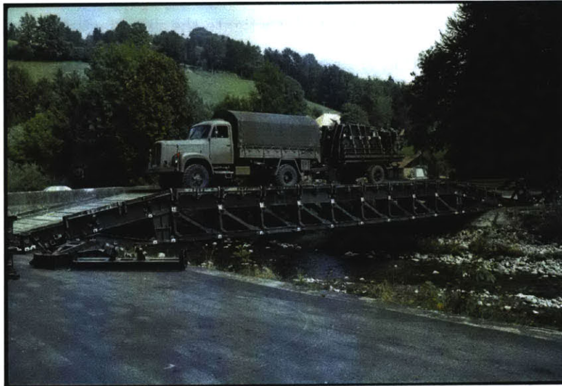
Figure 3-3: The Medium Girder Bridge being used by the Swiss Army [2].
