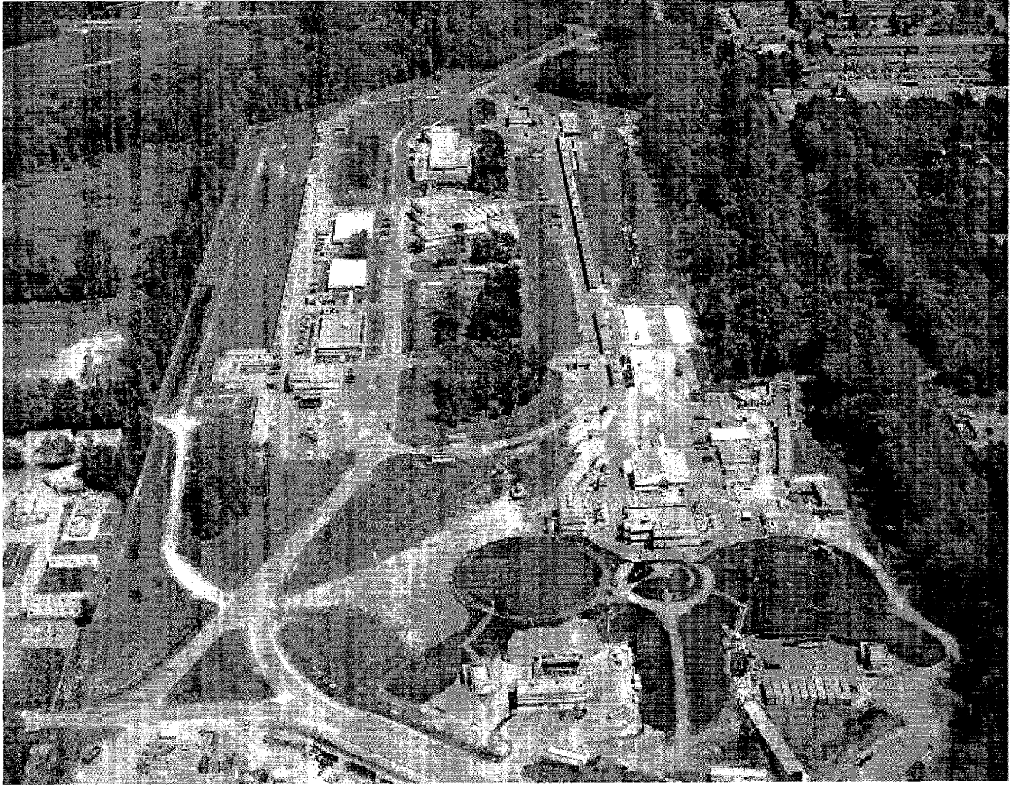
Figure 2-1: An aerial view of Jefferson Lab accelerator site and the three experimental halls.
