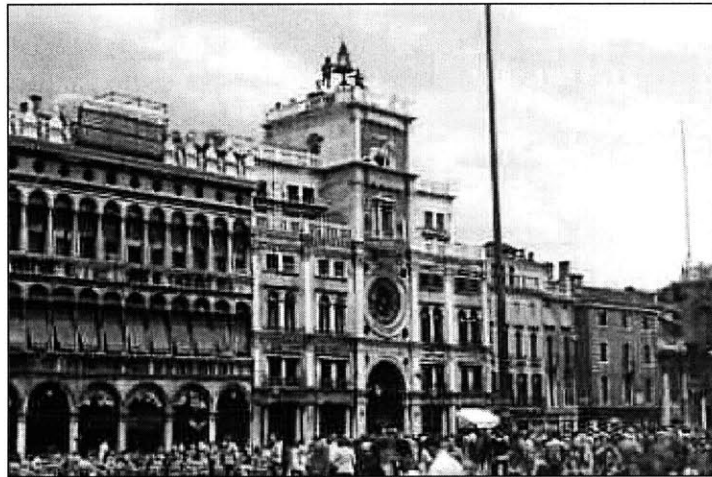
Figure 5. Tower of the Orologio. Source: Almesberger et. al. 2000.
