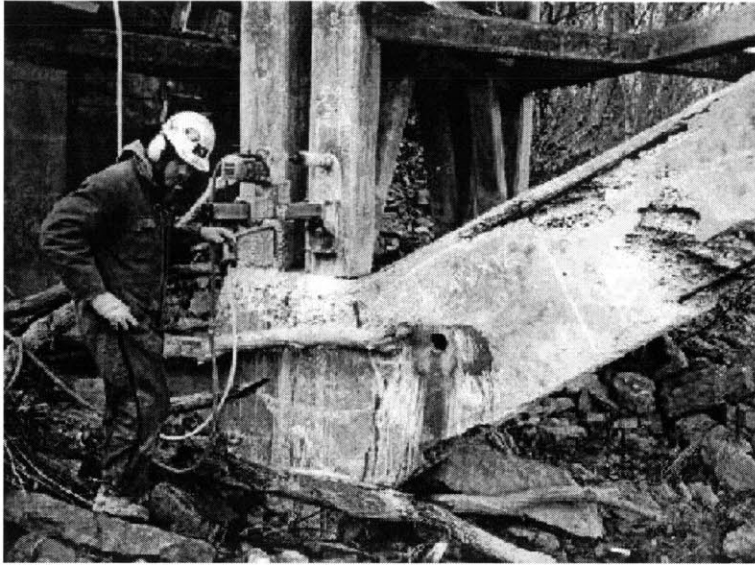
Figure 22. Coring at Putnam County Bridge. Source: Davis et. al. 2001.
