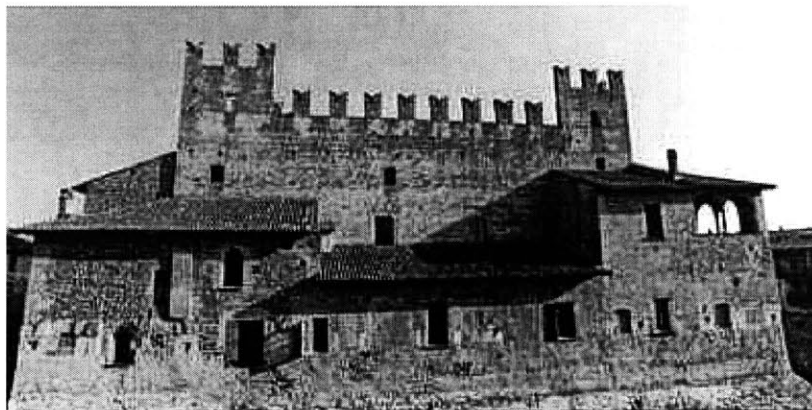
Figure 9. Malpaga Castle, front view. Source: Rosina et. al. 2000.
