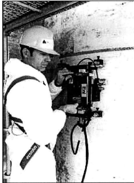
Figure 15. Inspector performing NDT tests. Source: Giunta et. al. 2000.
