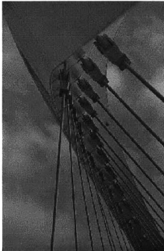
Figure 46: Connection of the cables to the arch in the Orleans Bridge
