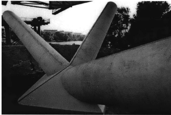
Figure 42: View of the tripod base of the Orleans Bridge
