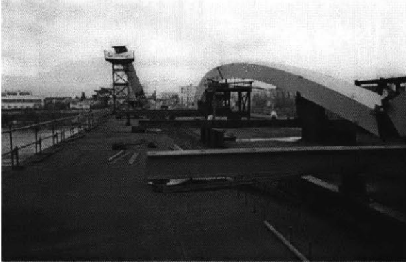
Figure 59: Arch elements on the Orleans Bridge deck
