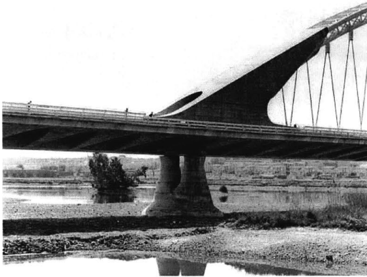
Figure 5: View of the twin piloti and the concrete abutment of the Lusitania Bridge
