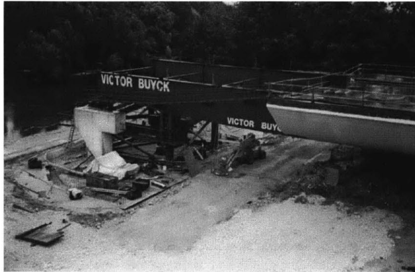
Figure 54: Launching nose of the Orleans Bridge
