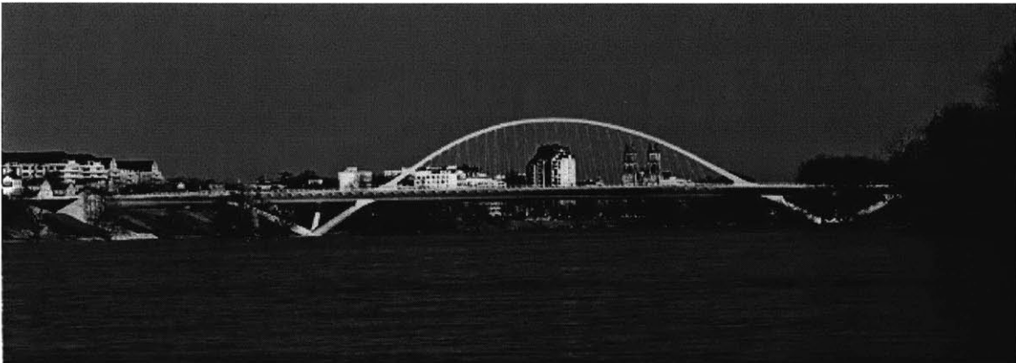
Figure 23: Overview of the Orleans Bridge
