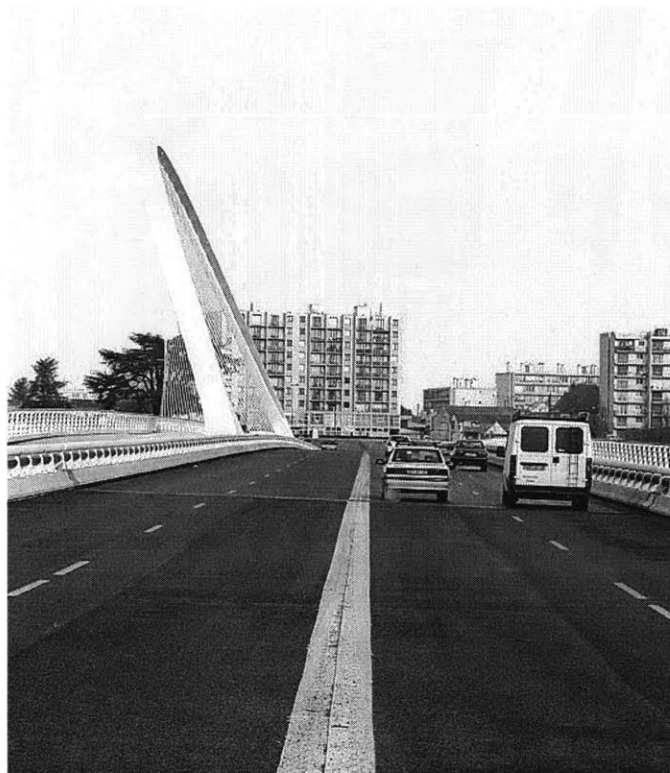
Figure 31: Orleans Bridge roadway
