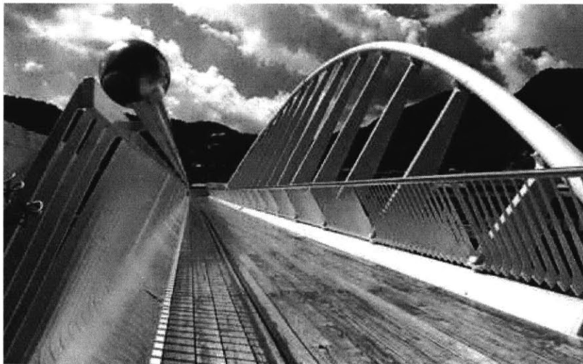
Figure 7: View of the walkway of the La Devesa Footbridge
