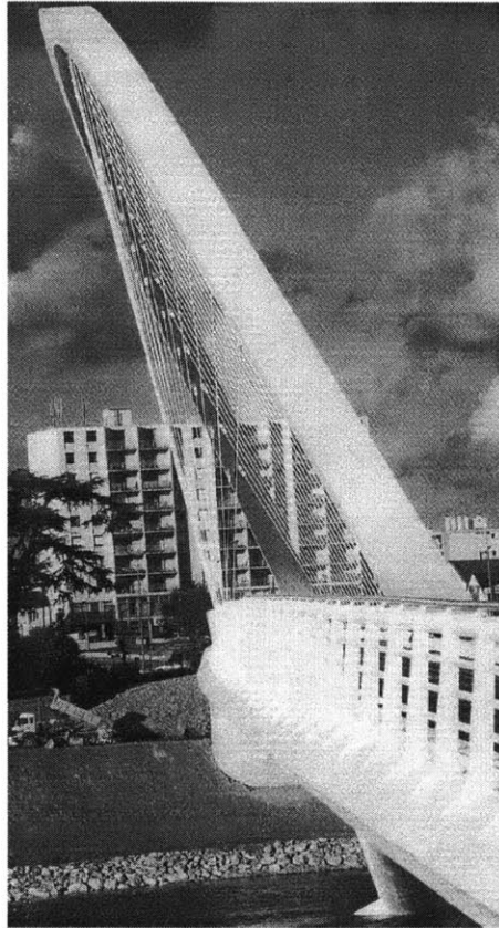
Figure 40: Hangers of the Orleans Bridge Note the masses attached to the cables
