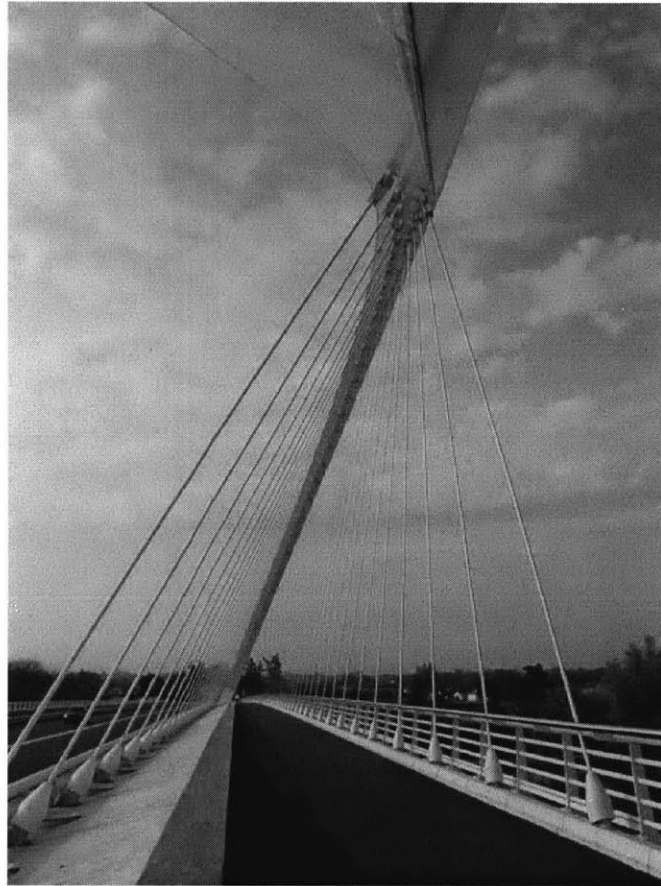
Figure 45: Orleans Bridge cables
