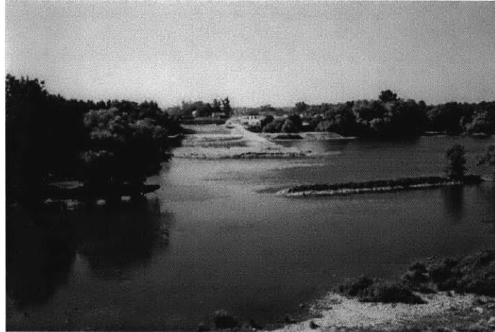
Figure 50: Overview of the site before the construction of the Orleans Bridge
