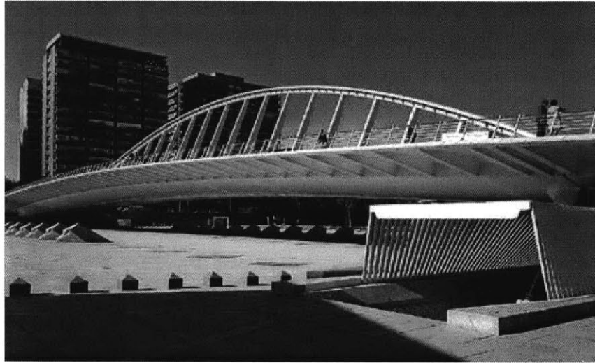
Figure 20: Overview of the Alameda Bridge with the metro entrance on the right
