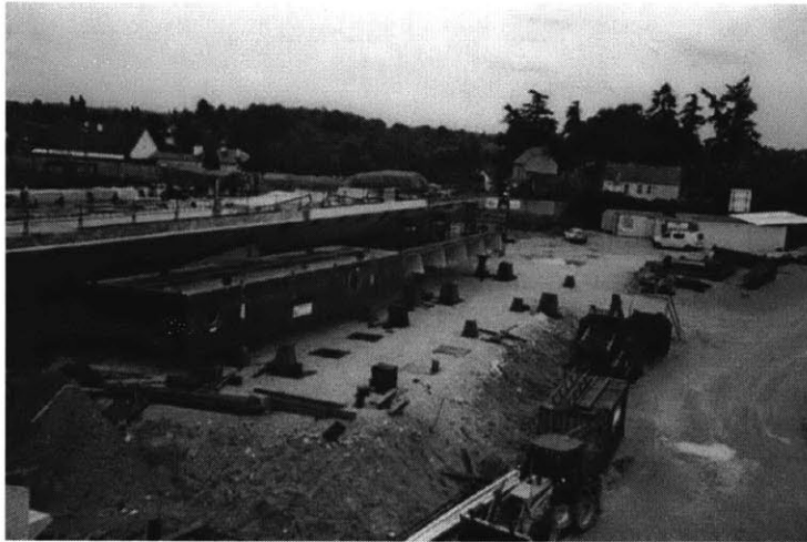
Figure 52: Assembly site of the Orleans Bridge located on the southern riverbank
