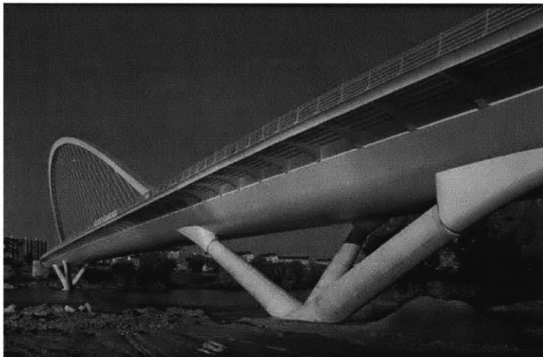
Figure 47: Southern tripod of the Orleans Bridge
