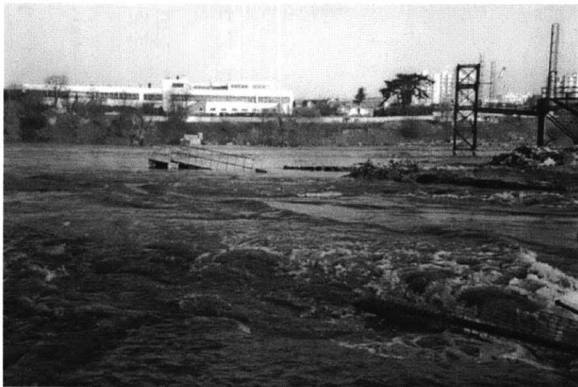
Figure 62: Floods of the Loire River during the Orleans Bridge construction
