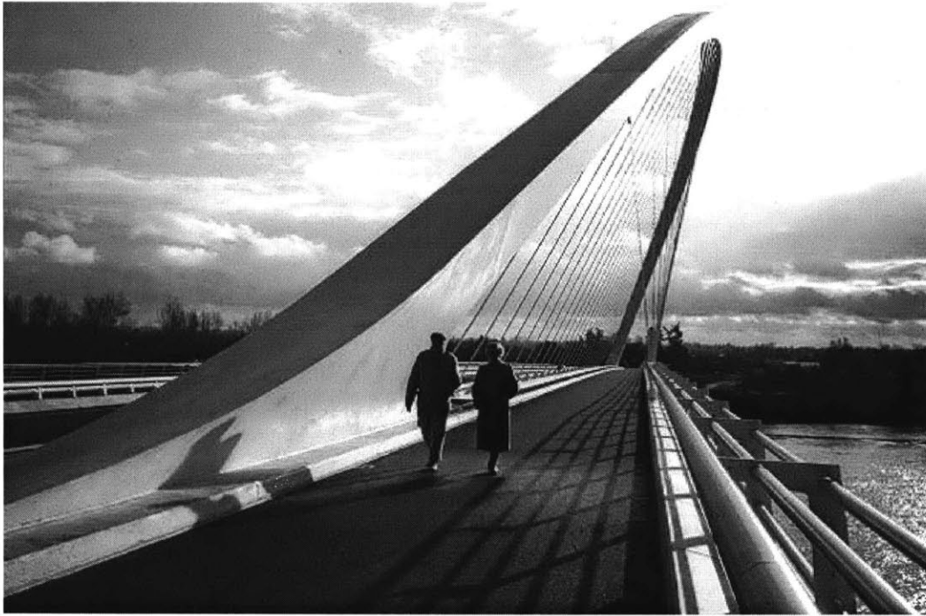
Figure 44: Orleans Bridge arch
