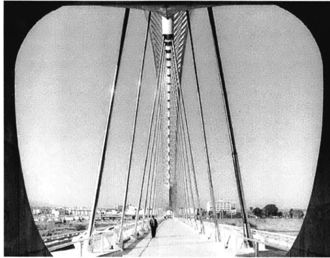
Figure 2: Central walkway of the Lusitania Bridge
