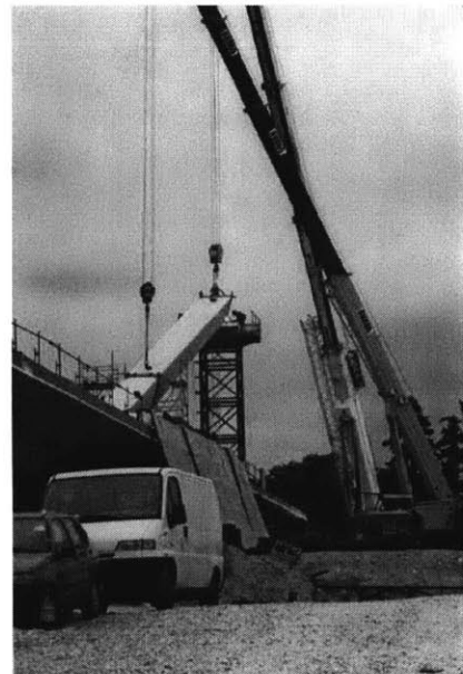
Figure 60: 400 tons mobile crane lifting an arch element of the Orleans Bridge
