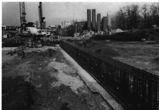
Figure 57: Concrete rails supporting the Orleans Bridge launching system
