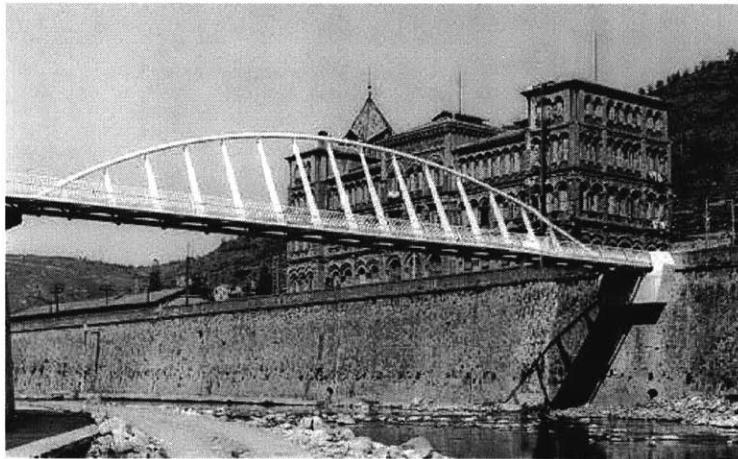
Figure 11: Overview showing the appendage on the right part of the La Devesa Footbridge
