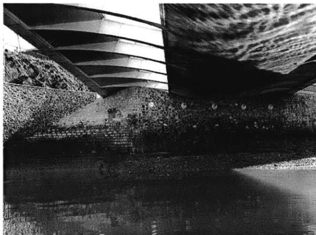
Figure 17: Separation between the main deck and the cantilevered pedestrian deck
