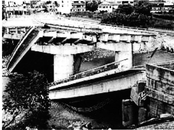
Figure 2-2: Unseating failure.
