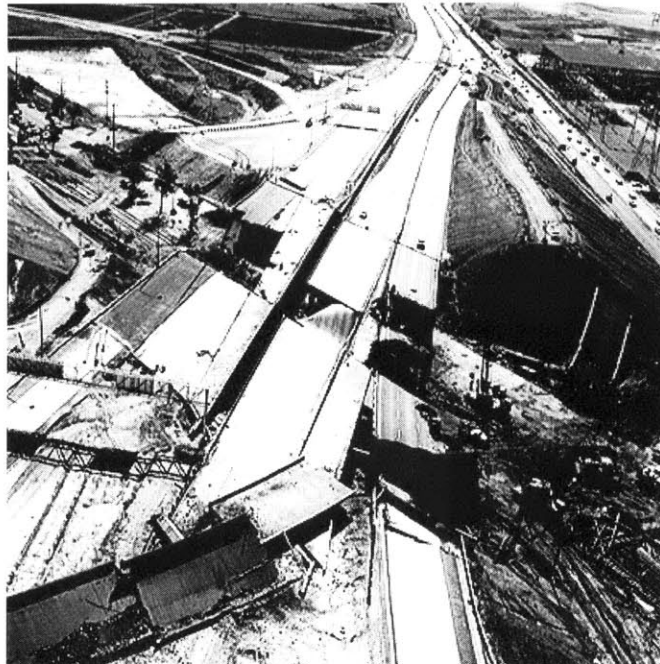
Figure 2-1: Severe seismic damage to highway bridge spans.
