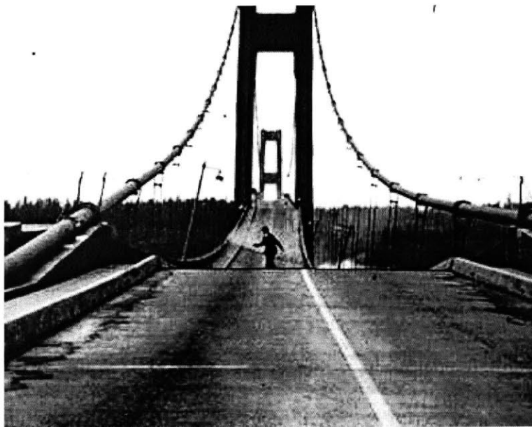
Figure 1 - 2: The collapse of the Tacoma Narrows Bridge
