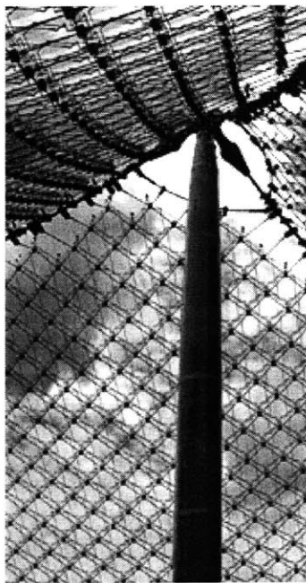
Figure 24: Connection between net and truss
