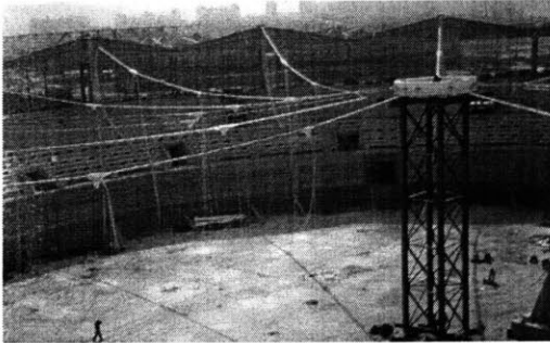
(a): Support tower placing tension ring into place.
