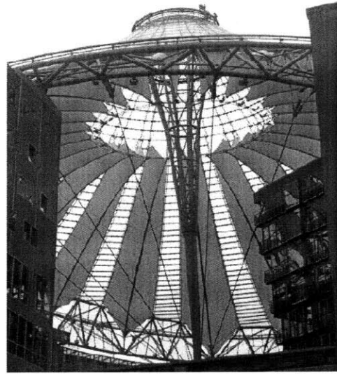
Figure 21: Roof of the Sony Center in Berlin
