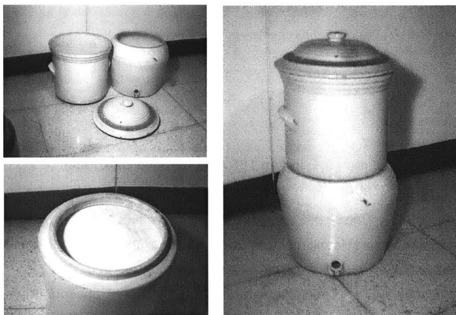
Figure 2.3: 100-Year Old Disk Filter from Spain
