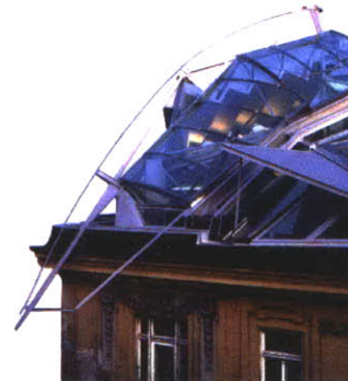
Fig. 1. "Rooftop Project" [Coop Himmelblau, Vienna 1988 - 1989 image source: http://www.ptutt.de/architectour/coophimmelblau-01.html ]
