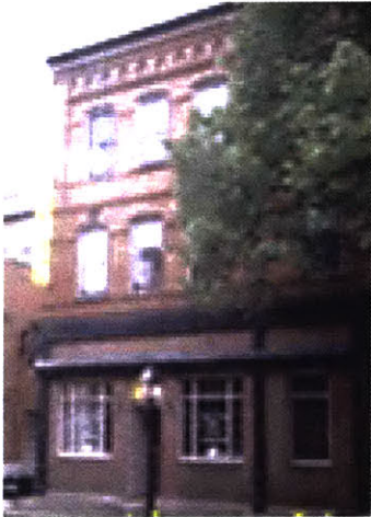
Kerrie Bellasario was able to convert this industrial building into a successful artist workshop: ARTWorks.
