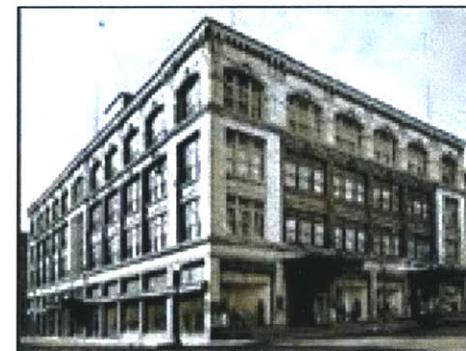
The old Star department store is now home to the University of Massachusetts at Dartmouth College of Visual and Performing Arts.
