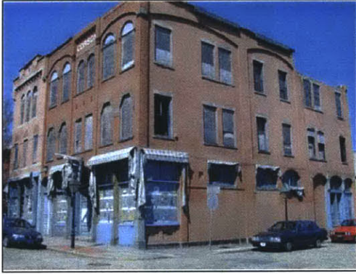
Many buildings still lie derelict in downtown New Bedford.
