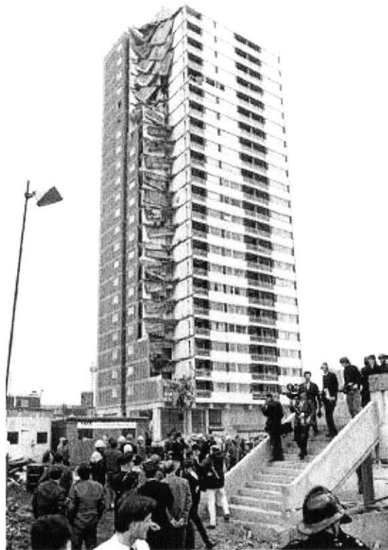
Figure 1: Ronan Point Failure (Rouse & Delatte)
