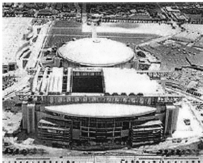
Figure 23: Reliant Stadium (foreground) under construction and Astrodome
