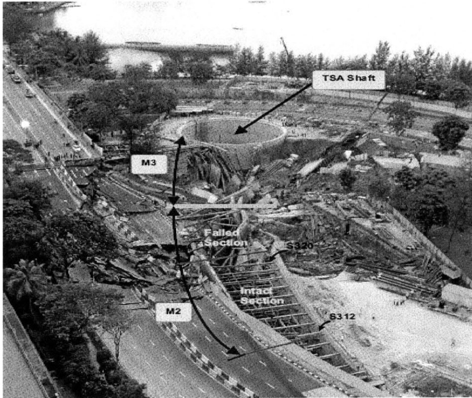
Figure 12: Site Before and After the Collapse (MOM, 2005)
