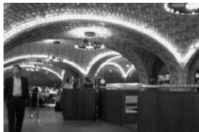
Fig.5.7. Guastavino vaulting in the "Oyster Bar", Grand Central Station in NYC.
