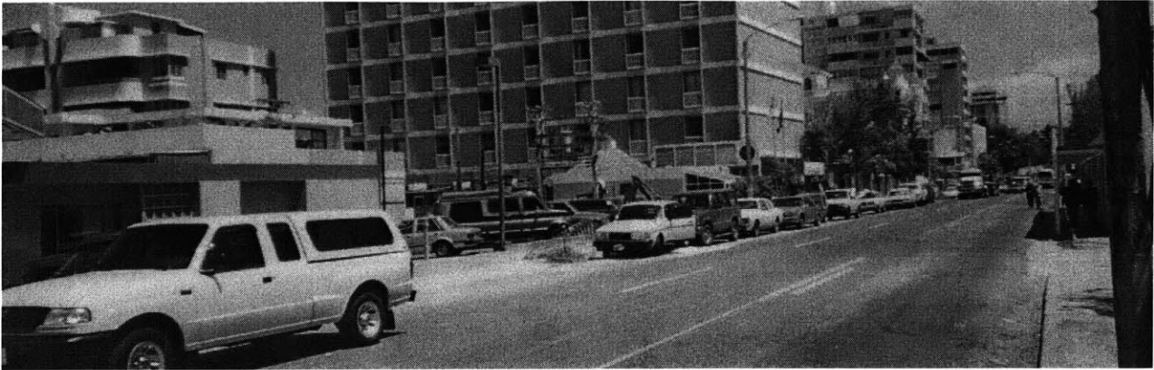
Figure 3-2: Multifamily housing along Munoz Rivera Avenue in Santurce. This is one of the more densely settled sections of the San Juan Metropolitan Area.
