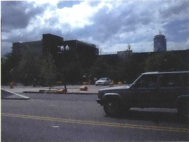
Figure 3.9 – Blackstone Elementary on Washington Street side
