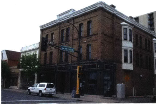
Figure 3.6 – GA Johnson Building
