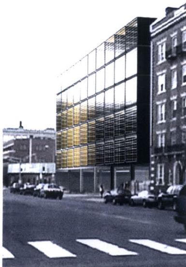
Perspective view of proposed development that uses OSB chassis and infill modules for customized residences.
