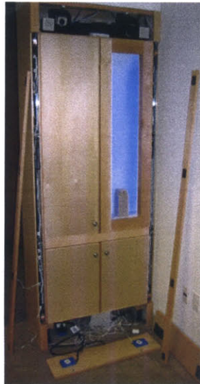
Access panels removed, power and data outlets at base of unit.
