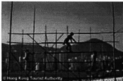
Figure 06: A worker on a scaffolding in Hong Kong
