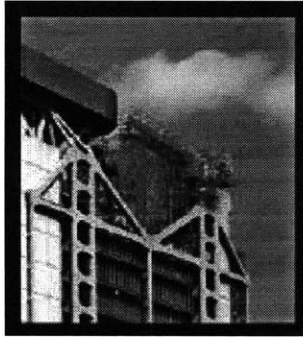
Figure 09: The Hong Kong - Shanghai Bank Building was built in large part using bamboo scaffolding
