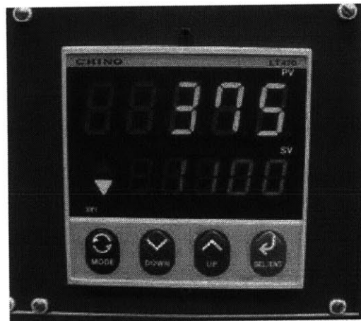
Figure 2.12: The controller displaying the actual and set temperatures.
