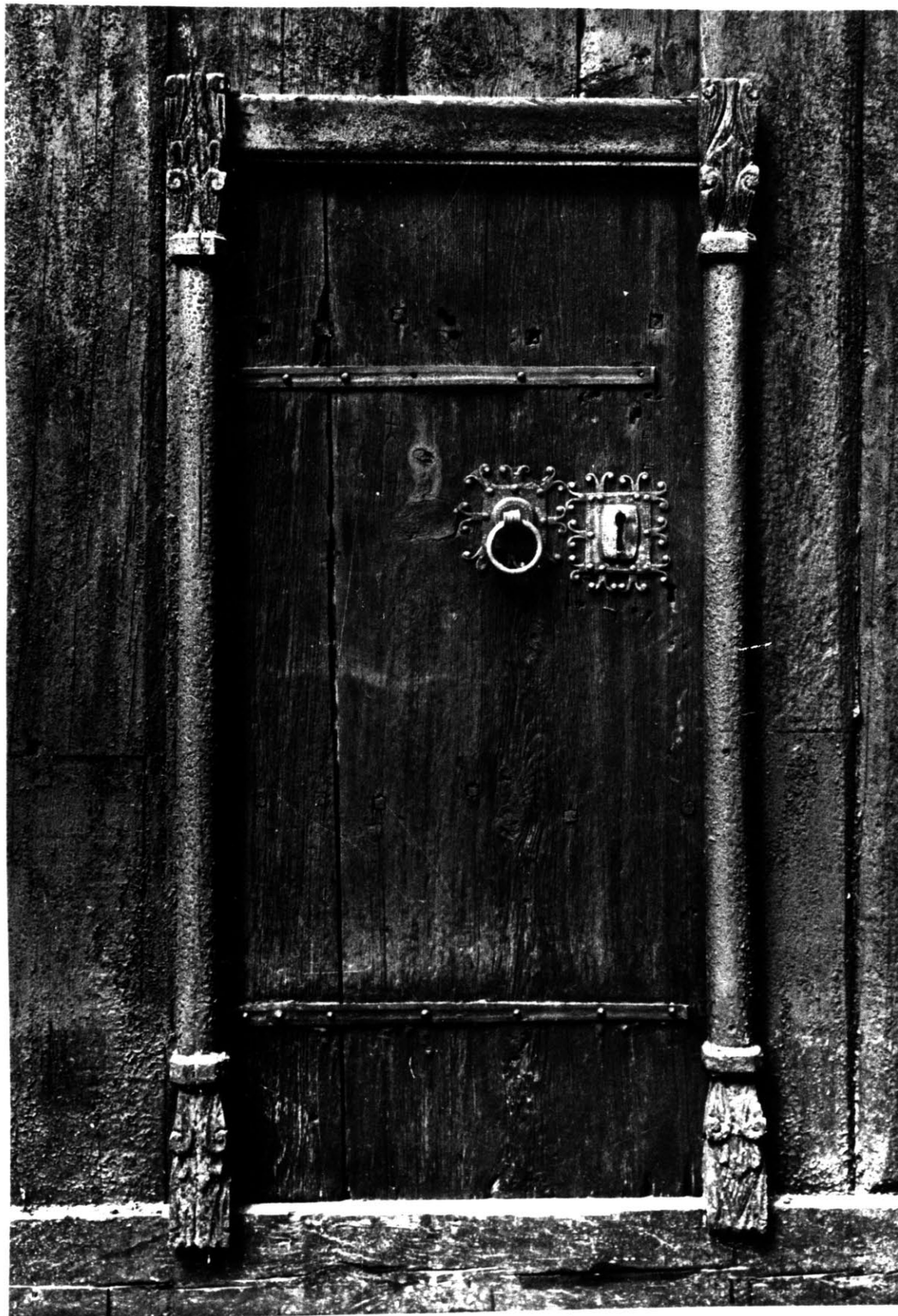
Door from the Garmo Stave Church
