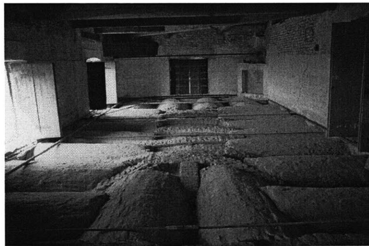
Fig. 4.13 Attic of Pojana above the side room without brick flooring exposing smaller vaults that are empty. Typically fill is placed over these followed by brick
