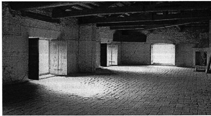
Fig. 4.12 Attic of Pojana above the side room with brick flooring
