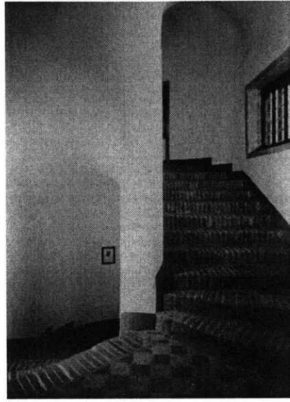
Fig. 4.26 Stairs at the Villa Cornaro - notice the vaulted ceiling supporting stairs above
