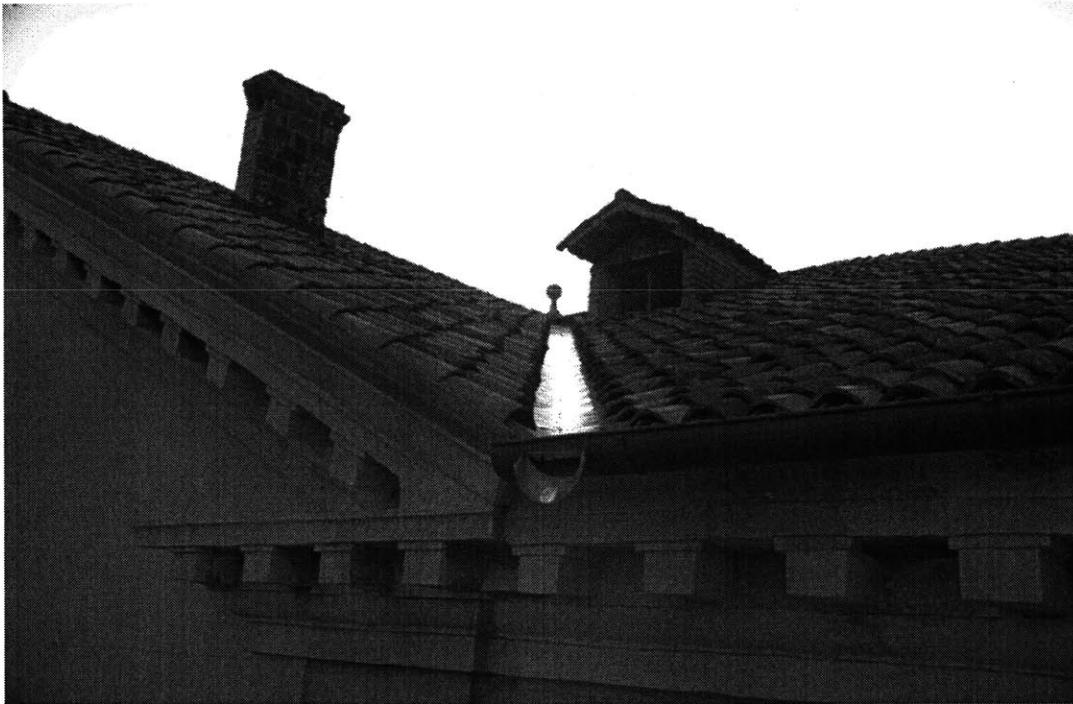
Fig. 4.47 Cornice and roof tiles at the Villa Pojana
