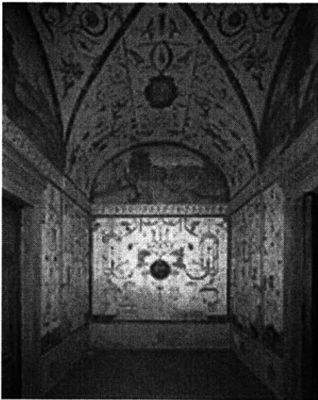
Fig. 4.16 Cross vault in back room of villa Pojana
