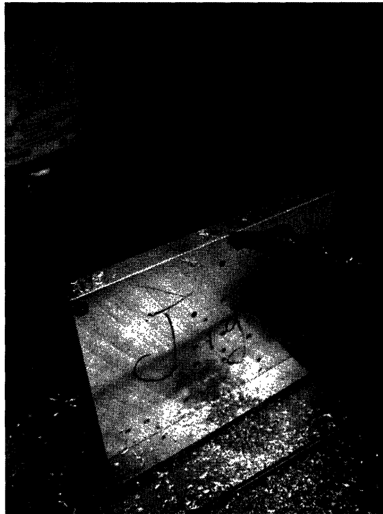
Fig. 8. Drilling the holes in the middle plate for the O-ring rods.
