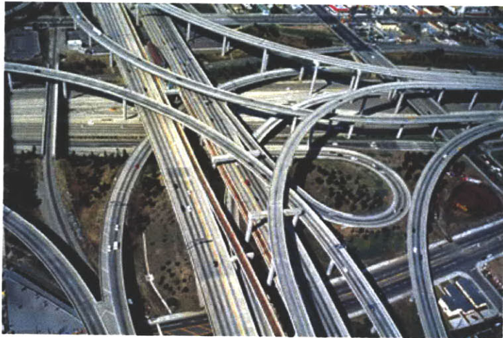
Figure 5.4-2 Aerial View of Harbor Freeway
