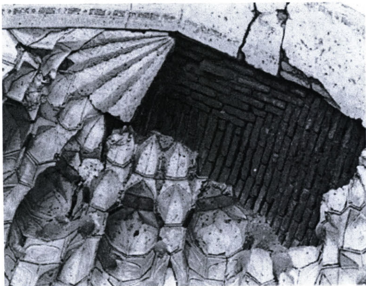
Fig. 11. (above) Madrasa of Saray Mulk Khanum, muqarnas suspended from brick structure.
