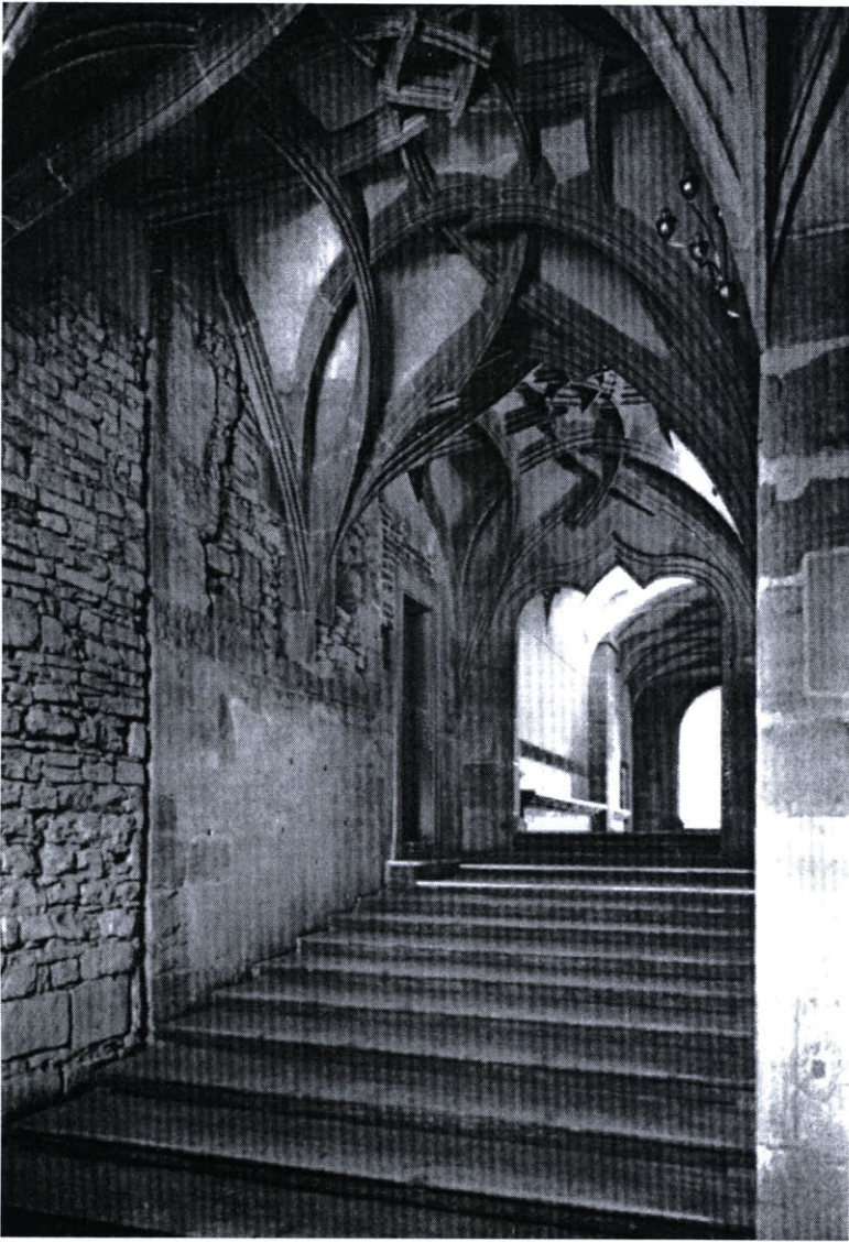
Fig. 6. Rider's Stair at Prague cathedral.
