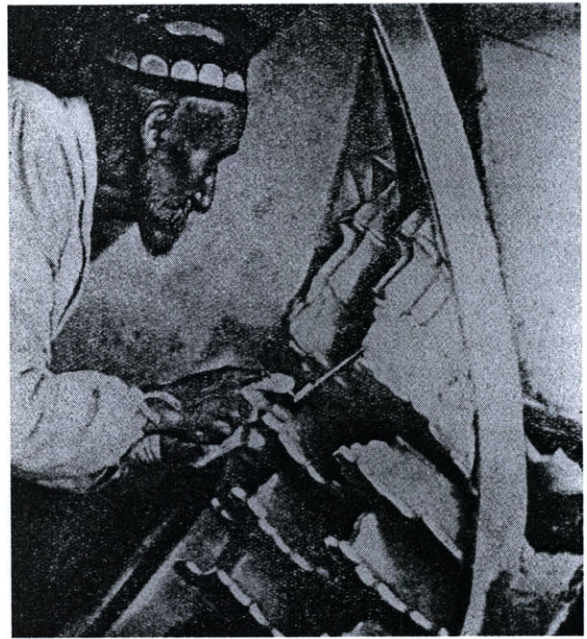
Fig. 10. The craftsman filling in the vertical modules of muqarnas.
