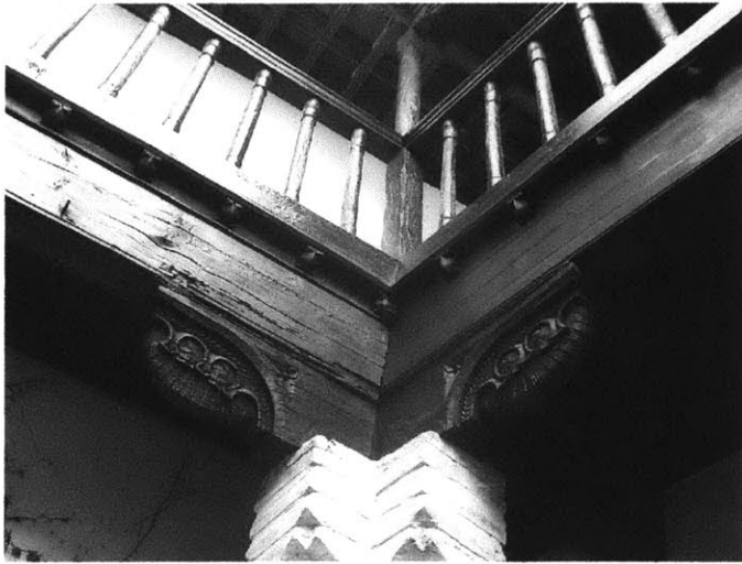
Figure 6. Wooden gallery supported by brick column. Note ornate carvings.
