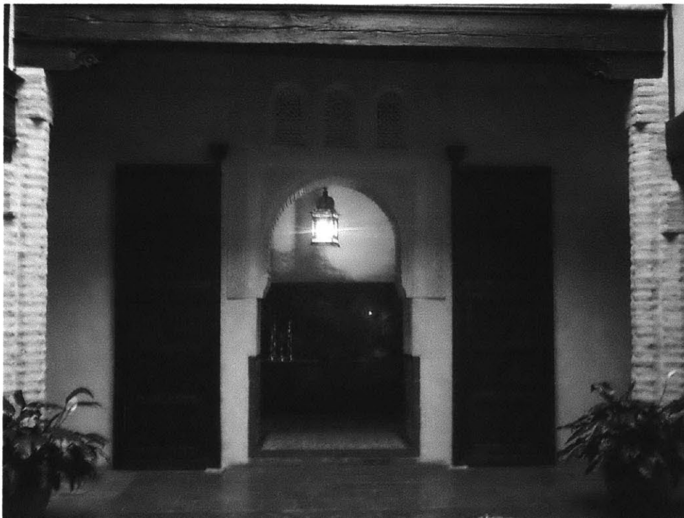
Figure 8. Vanos windows, plaster carved arch, and brick columns
