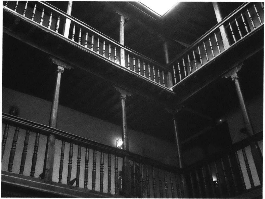
Figure 9. Example of wooden balustrade, columns and corbels with ornate carving
