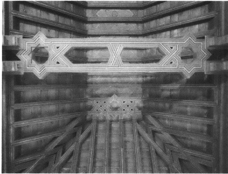
Figure 13. Woodwork of the ceiling
