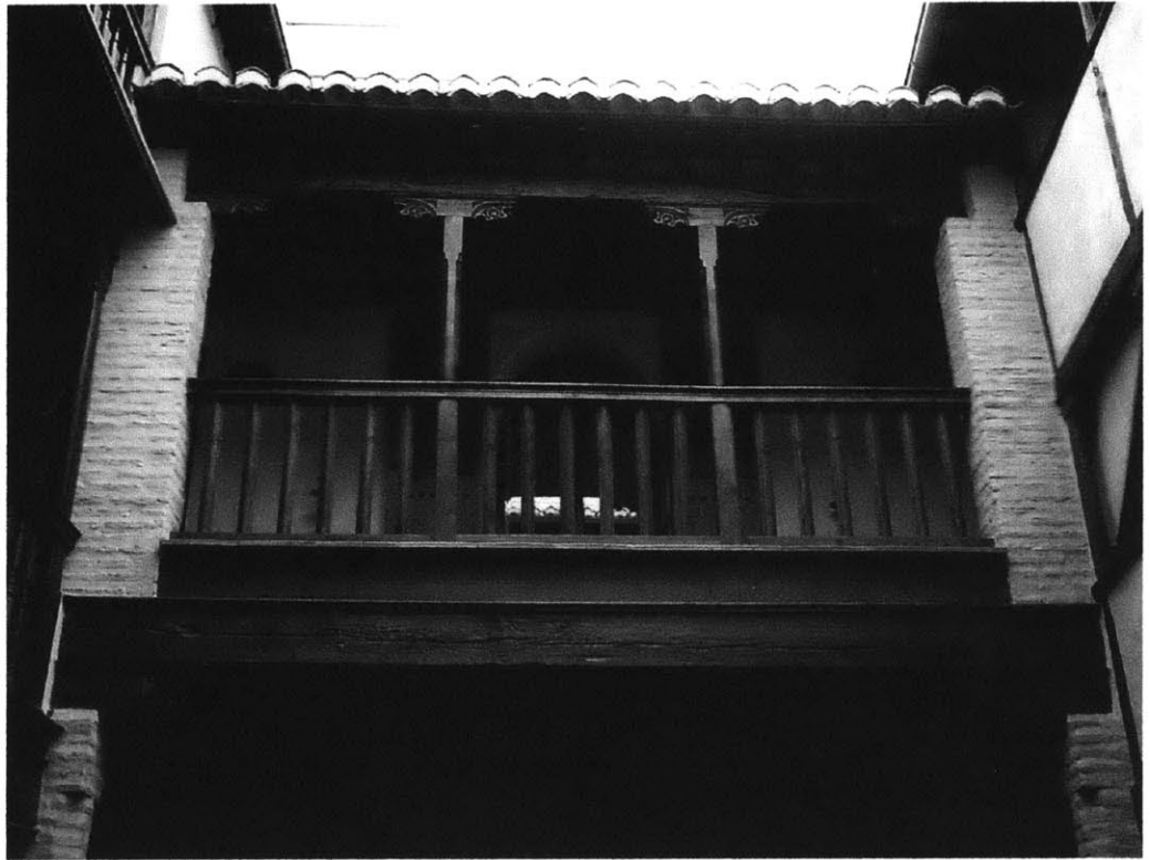
Figure 10. View of masonry support elements and wooden balustrade with carved corbels
