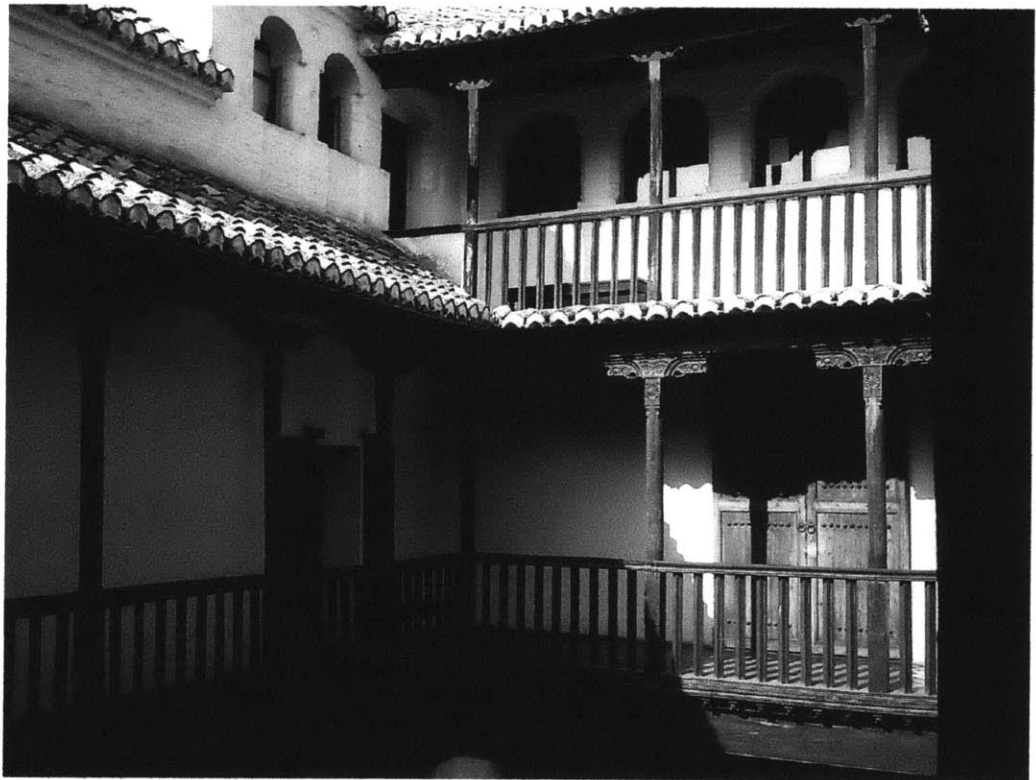
Figure 10. Another example of carpentry in the galleries
