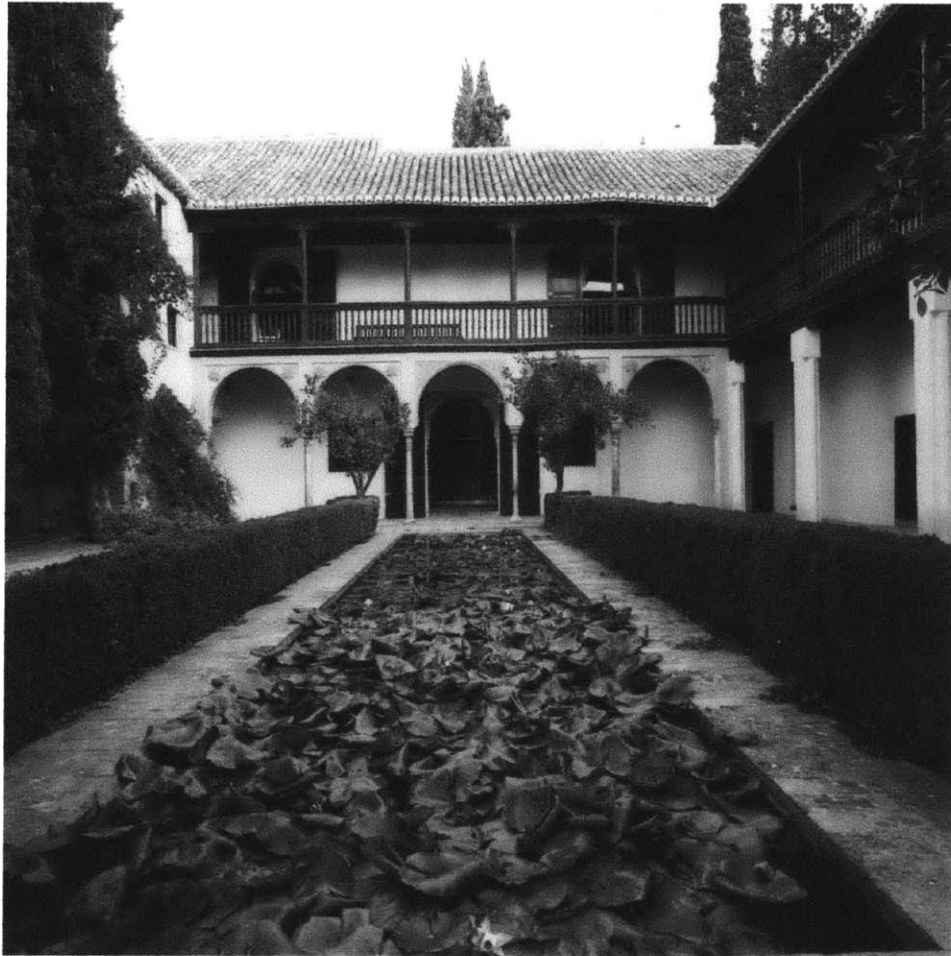
Figure 4. Patio of rear house of the Casas del Chapiz. Note the five arches..
