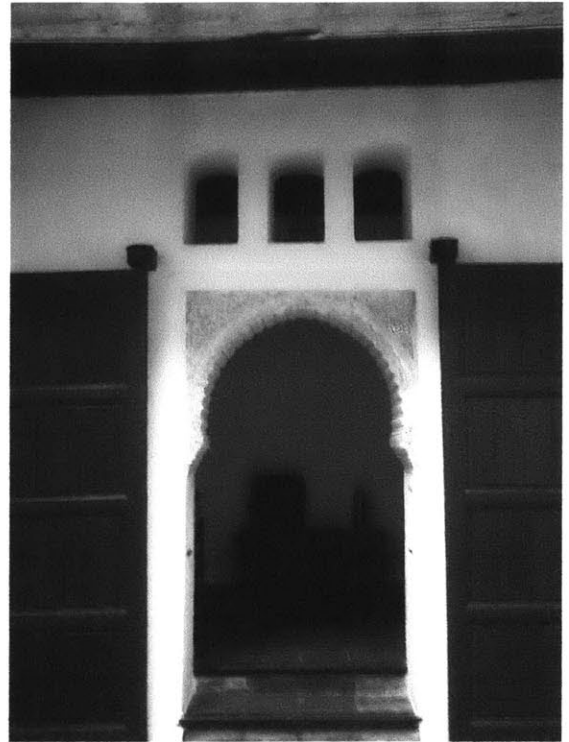
Figure 7. Vanos windows over the door to the main salon
