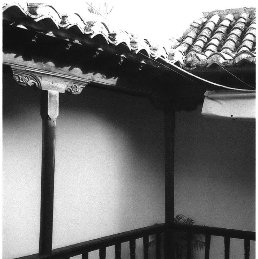
Figure 11. Columns, corbels, and tiled roof
