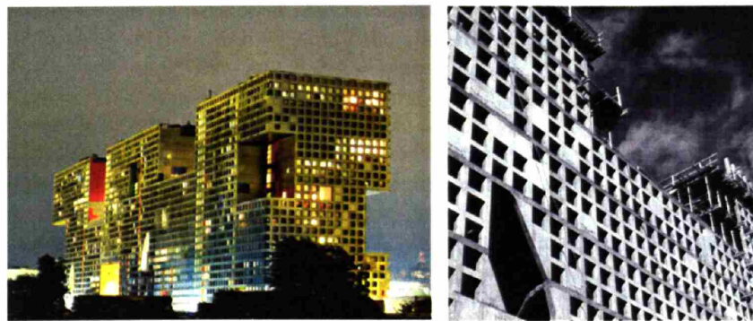
Figure 2. Simmons Hall undergraduate residence, MIT: View from Vassar Street, and exterior view of the "perforated" structure during construction
