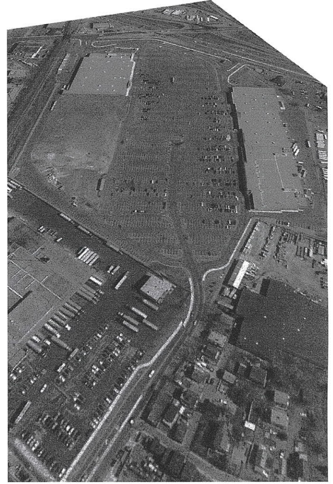
The South Bay Shopping Mall
