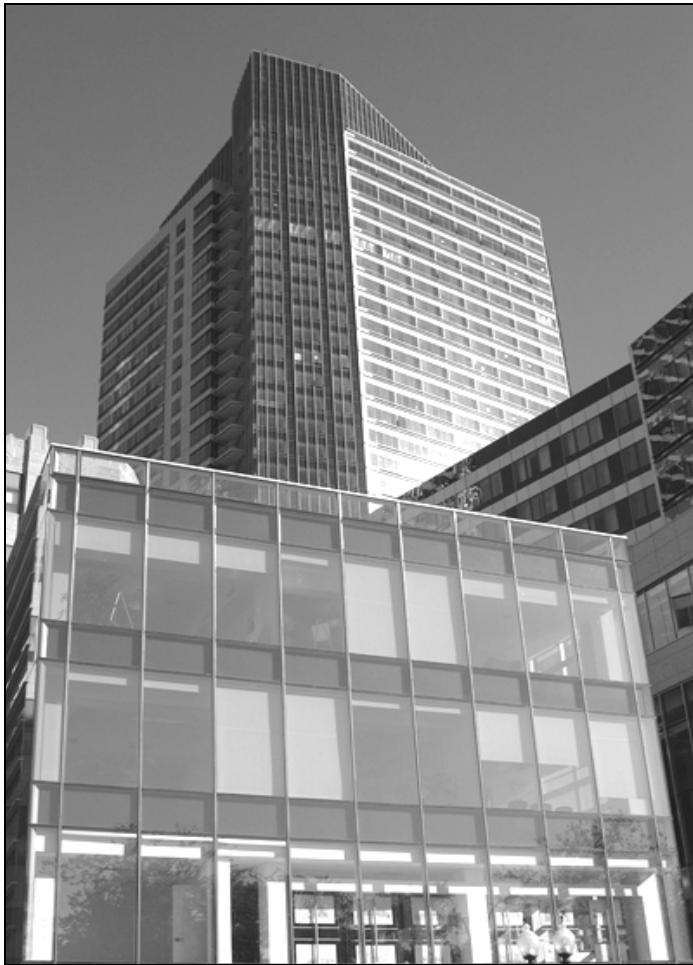
Figure 4.2.3: Façade at Street Level
