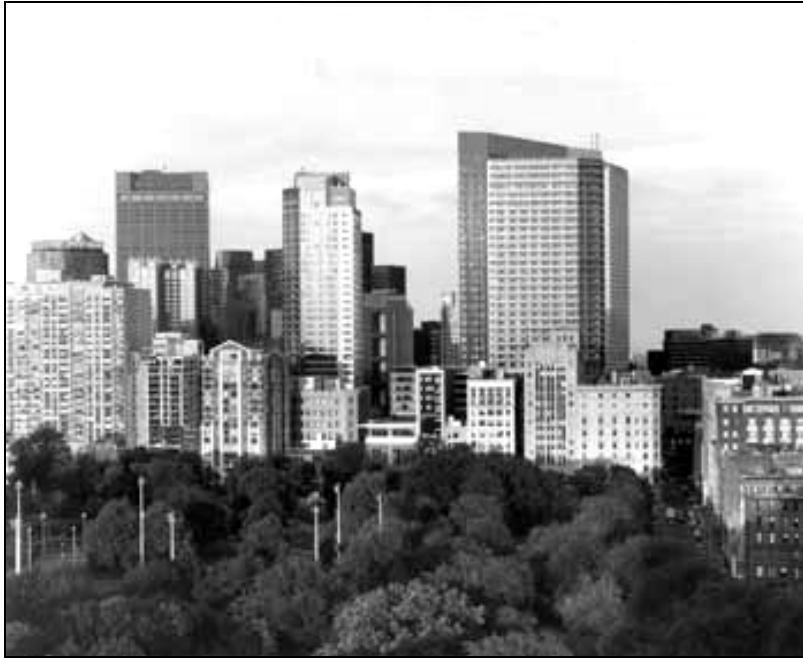
Figure 4.2.2: Aerial View of Towers
