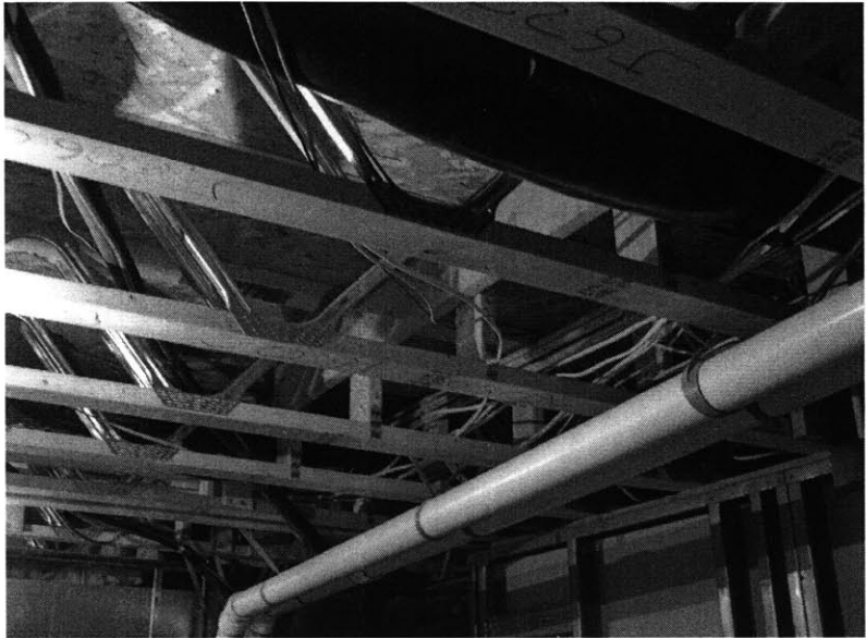
Figure 4.13 Open Web Floor Joists (note electrical wiring)
