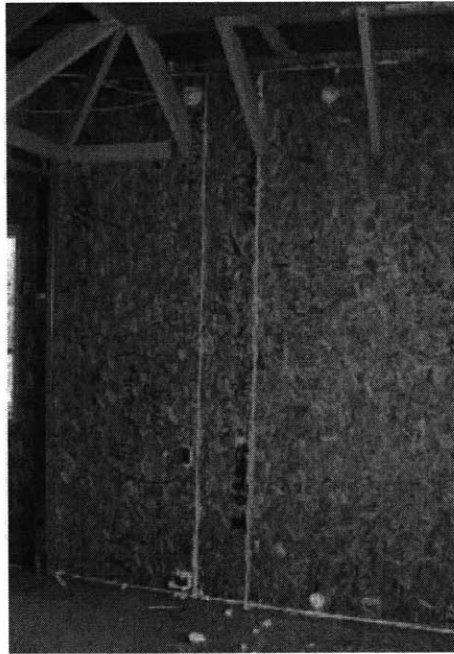
Figure 4.15: SIP Sealing (white caulk on SIP interior)
