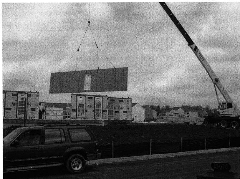
Figure 4.16: The New Framing Paradigm (Pulte subs assembling walls)
