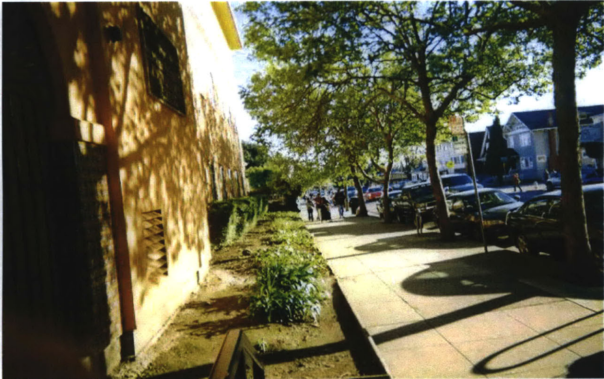
Unity Council Building
