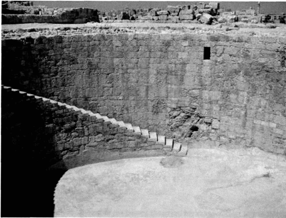
Figure 41 Cistern at the Amman Citadel (Photograph Conrad Schmidt)
