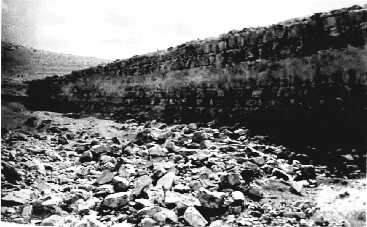
Figure 17 The South-East Dam of al-Qanatir. This is one of two massive stone dams located in central Jordan dating to the Umayyad period. These dams were used to collect and store rain water that was used to irrigate the qusur . (Photograph by Conrad Schmidt)
