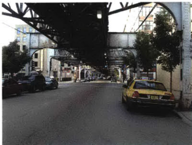
OVER-STREET STRUCTURE PREDOMINANT IN THE STREETScape
