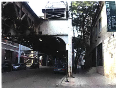
EXQUISITE ELEVATED STRUCTURES
