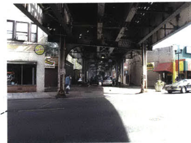
"GAP" ON LINCOLN AVENUE
