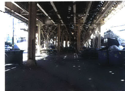
CLUMSY SPACE UNDER THE TRACKS
