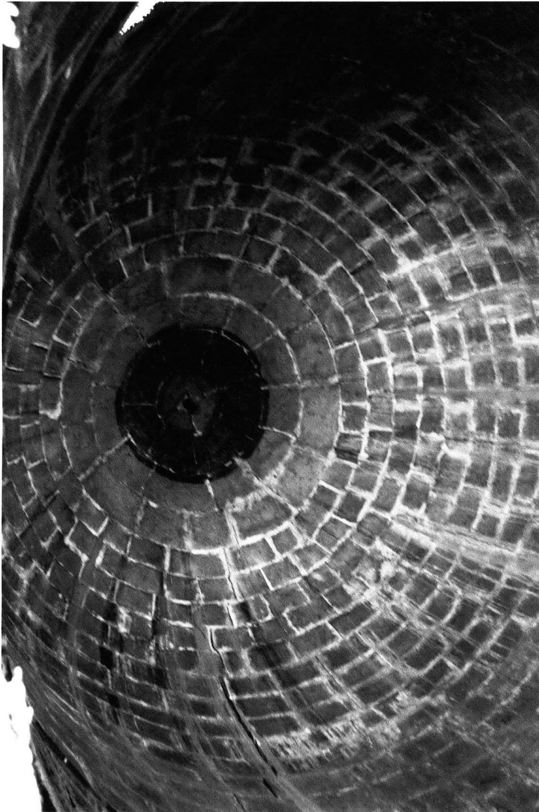
Fig. 2.3 Interior of the Mausoleum of Umm Sultan Sha'ban. The ashlars constituting the rings are very evident also in the interior. Photo by the author
