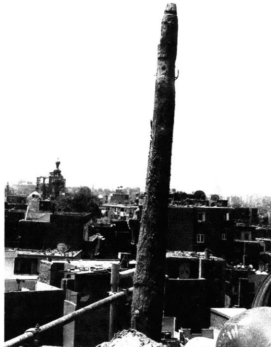
Fig. 2.4 Restoration work at the Mausoleum of Umm Sultan Sha'ban. The pictures show that the crescent is hollow and it is held by a wood post that is embedded in the dome top part. Photos courtesy of the Aga Khan Trust for Culture
