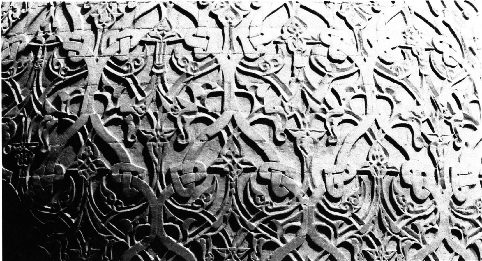
Fig 2. 27 Detail of the doem decoration. The wood pegs used during construction are visible in correspondence of the joints.
