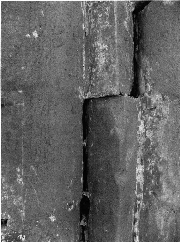
Fig. 2.6 Restoration work at the Mausoleum of Umm Sultan Sha'ban. The pictures show the external and internal step-like cracks. Photos courtesy of the Aga Khan Trust for Culture
