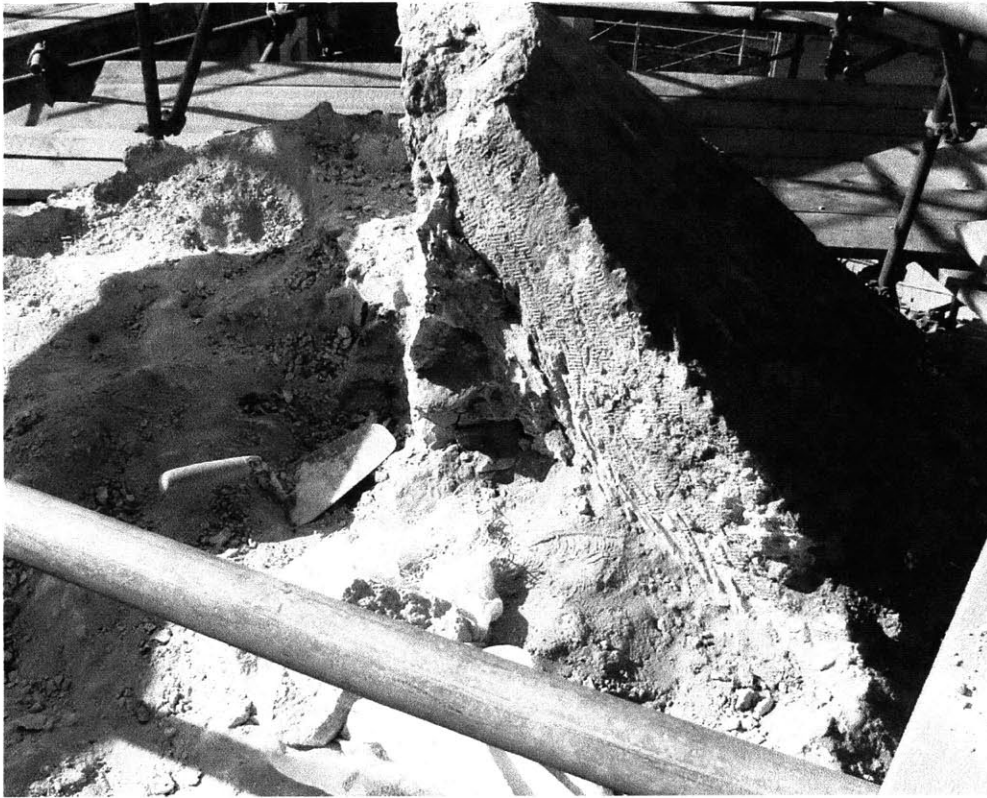
Fig 2.29 a,b, The restoration of the upper part of Khayer Bek dome shows the stone blocks covering the hollow inside filled in with rubble. Pictures courtesy of the Aga Khan Trust for Culture.
