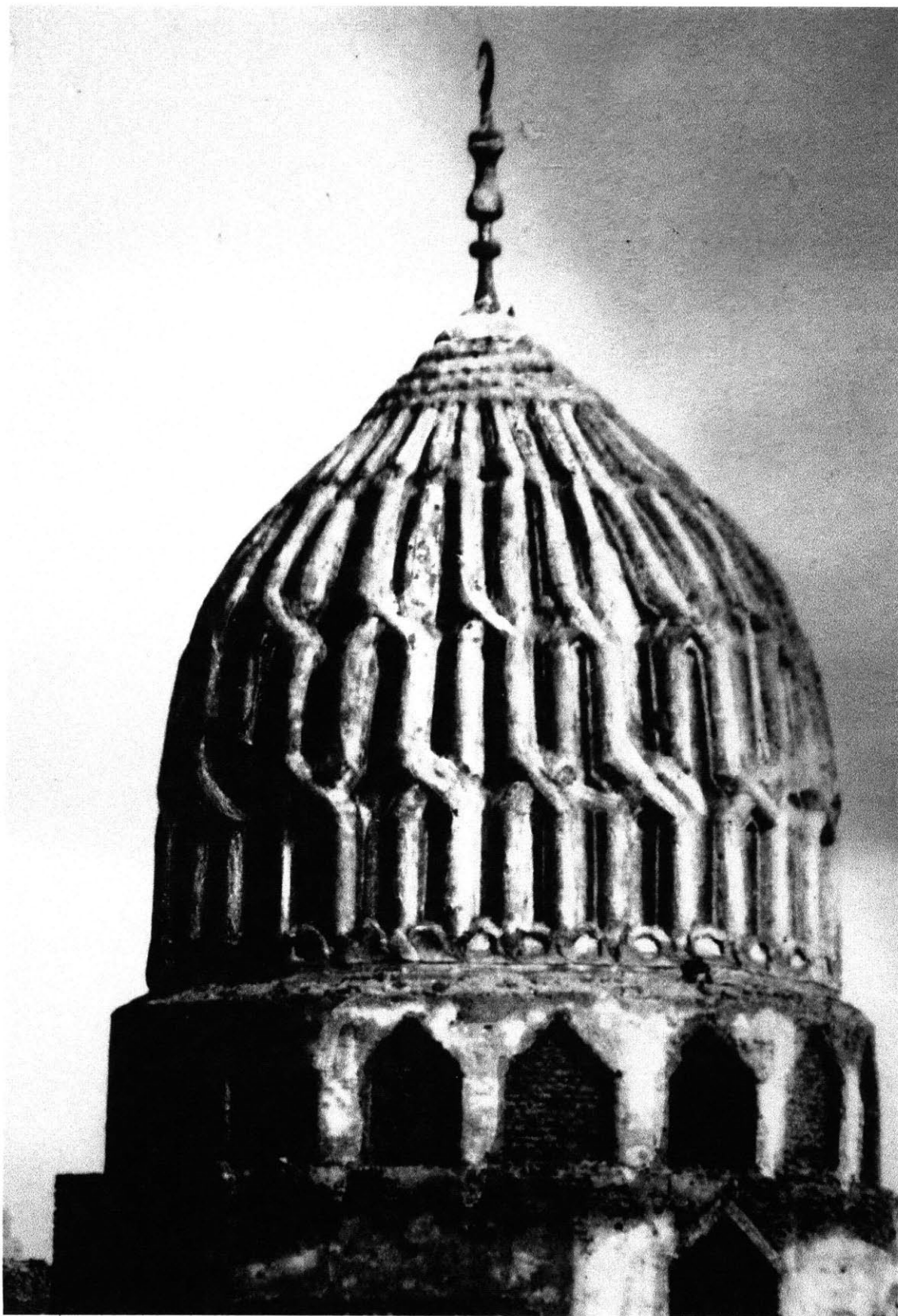
Fig. 1.16 Mausoleum of Khadiga Umm al-Ashraf 1430-1440 A.C. © Creswell Archive, Ashmolean Museum, neg. Image courtesy of Fine Arts Library, Harvard College Library
