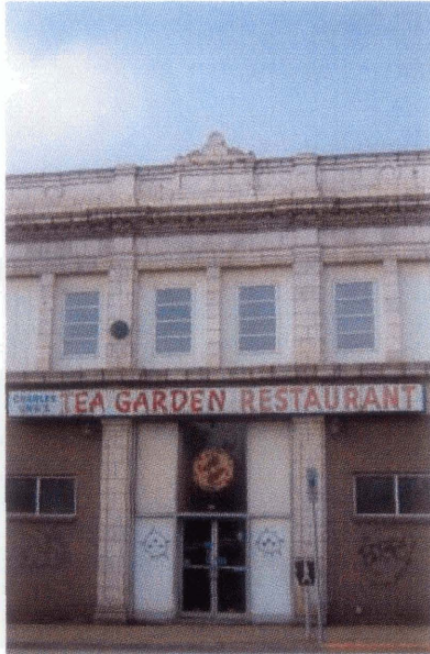
Empty properties in East Liberty's commercial core
