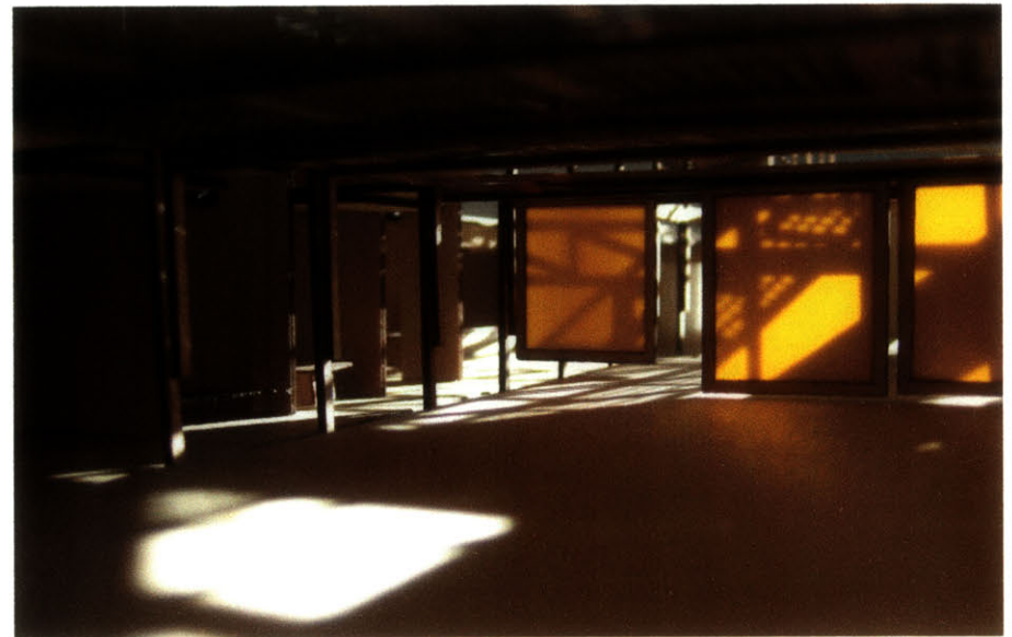
Dividing panels at the workshop area. The translucent panels are hung from the screen (infra)structure and allow the communal public space to be segmented and adapted for multiple uses, but still preserve a degree of overlap through light and small apertures.
