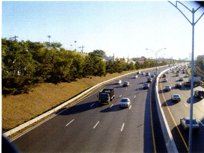
Fig. 78. View of the Site
