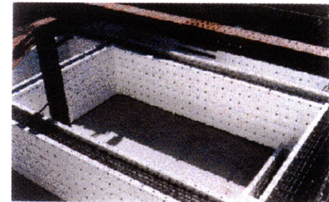
Fig. 35. INSULATION FORMWORK. Formwork left in place after casting as insulation.
