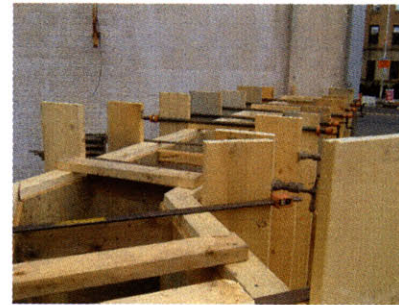
Fig. 71. Image of Formwork 2.
