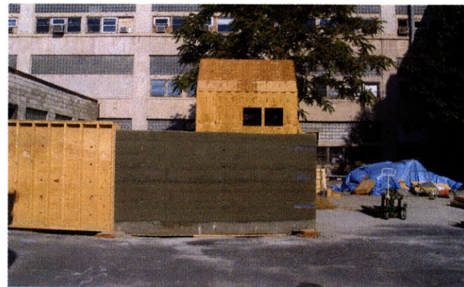
Fig. 72. Image of The Wall. Made using formwork 1.
