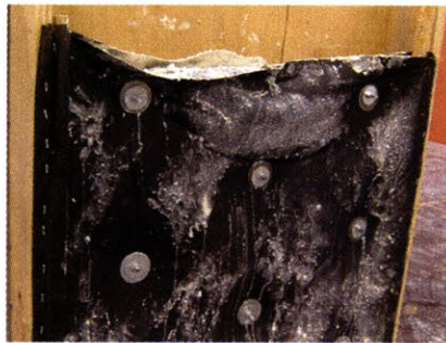
Layers are separated and fabric removed.
