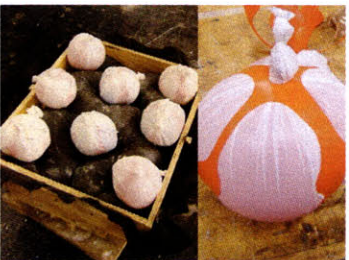
Ballons attached to formwork with hollow tubes
