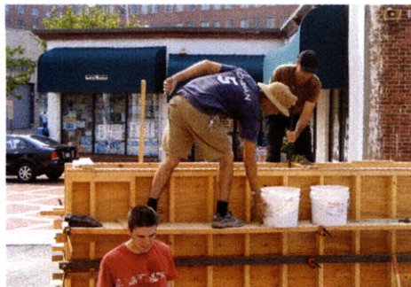
Fig. 69. Construction Image. Horizontal support is used as footing for the workers.
