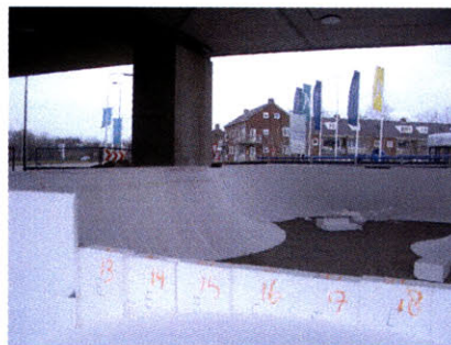
Fig. 37. Skate Bowl Construction Using Foam.
