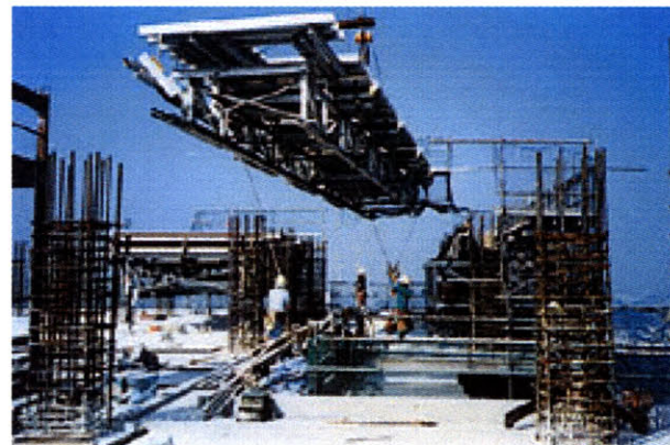
Fig. 46. OMNIA DECK PLATE FORMWORK.
