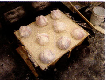
Concrete poured halfway up the ballons
