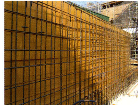
Fig. 51. WALL FORMWORK.
