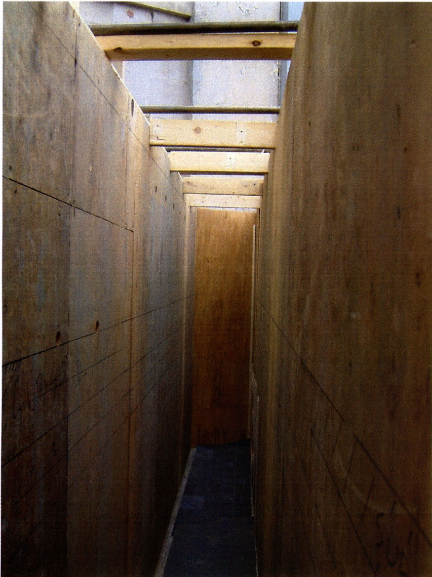
Fig. 73. Inside of Formwork 2. Space is free of pipe clamps.
