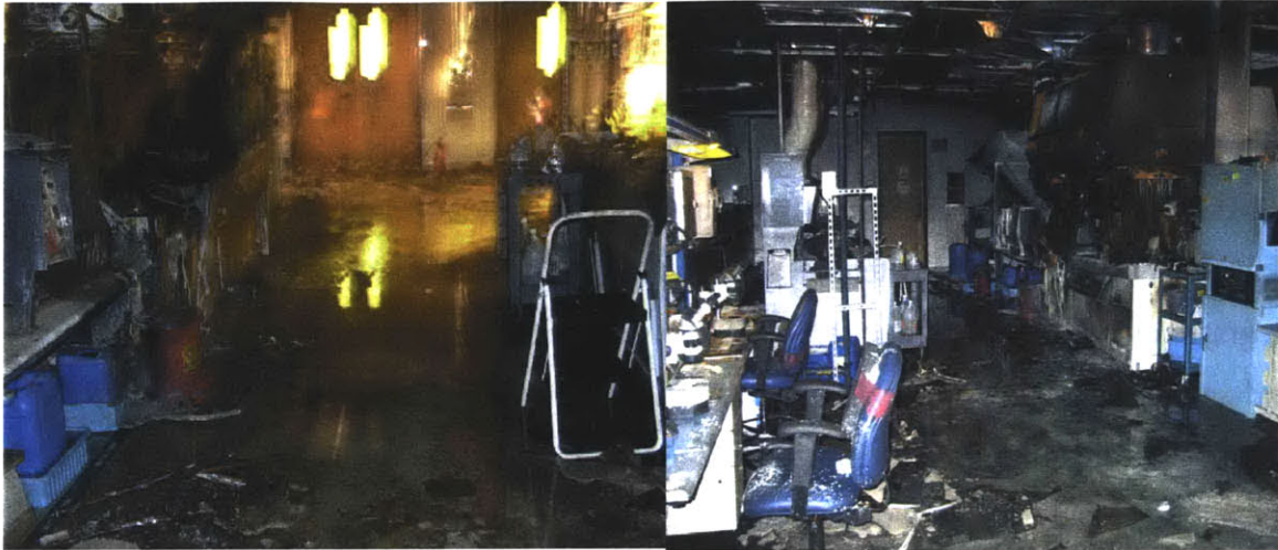
Figure 1: Aftermath of Fire
