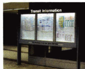
Figure 3-5: This CTA information kiosk may prevent customers confined to wheelchairs from seeing the fine print on some devices.
