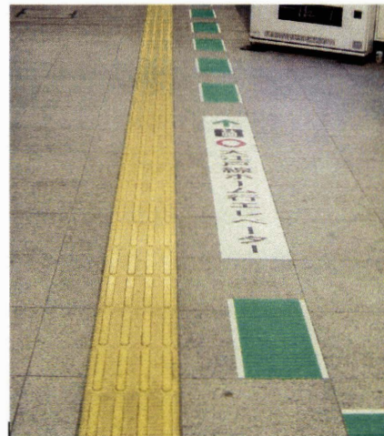
Figure 4-31: An example of tactile directional elements in a Japanese subway station. (Courtesy of Jeffrey Sriver)
