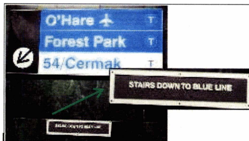
Figure 5-44: This tactile directional device at Clark/Lake does not include the arrow provided for sighted passengers.
